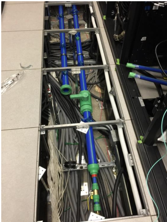
Cooling Line Installation
