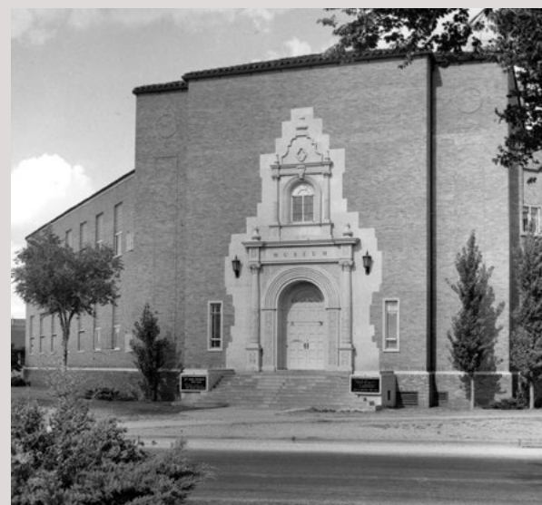
Appearance of the Museum after completing the initial construction, ca. 1949 Courtesy of Southwest Collection/Special Collections Library, Texas Tech University
