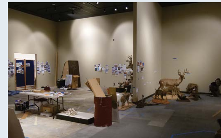
Early stages of construction in the new Biodiversity exhibit.
