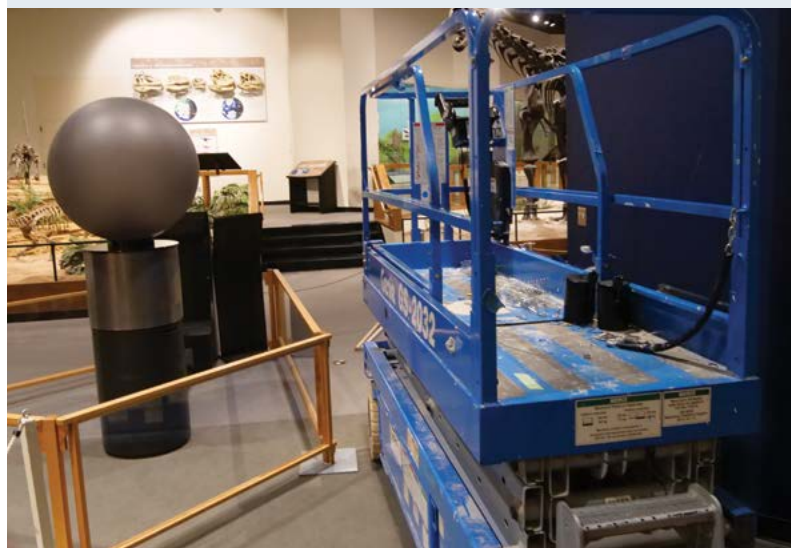
Construction underway in the Changing World gallery.
