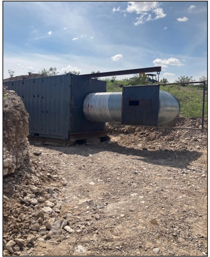
The assembled structure before burial, showing the metal culvert that serves as the entry tunnel, the shipping container that serves as the cave, and the entry door that can be adjusted depending on the season.
