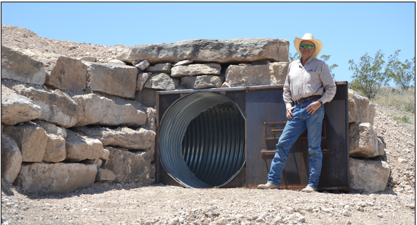
General Manager Billy Pat McKinney at the entrance of the completed bat cave on the property of the El Carmen Land and Conservation Company.
