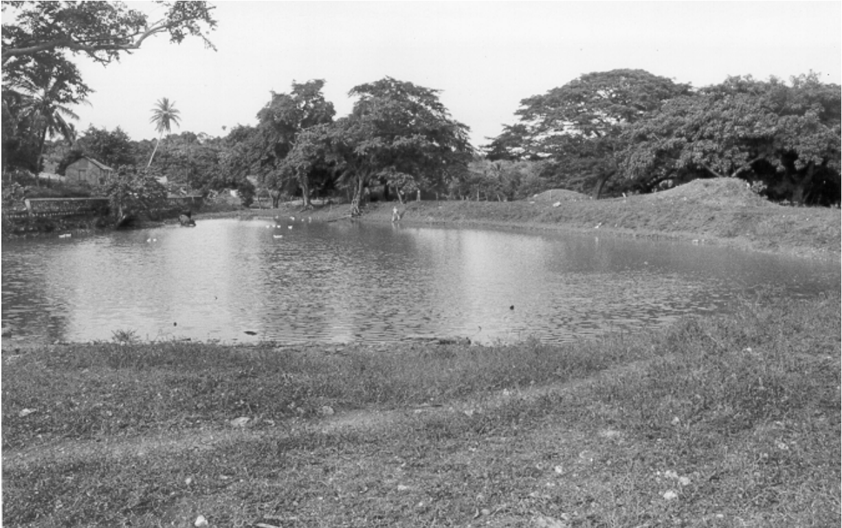
Figure 4. A view of the earthen tank at Queenhythe, St. Ann Parish, Jamaica.
