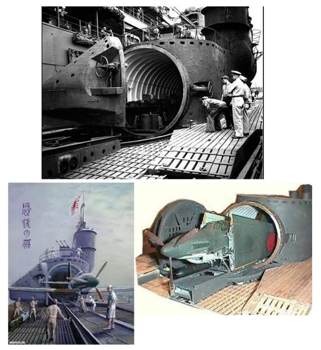
(Top) U.S. Navy photograph of captured Sentoku submarine. This view shows the open hatch for the aft end of the seaplane hangar mounted on the top deck mid-line.
