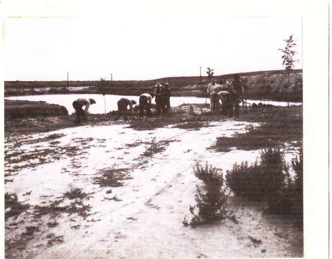
Detail of the reservoir at ground level with the work crew ca. 1930s.
