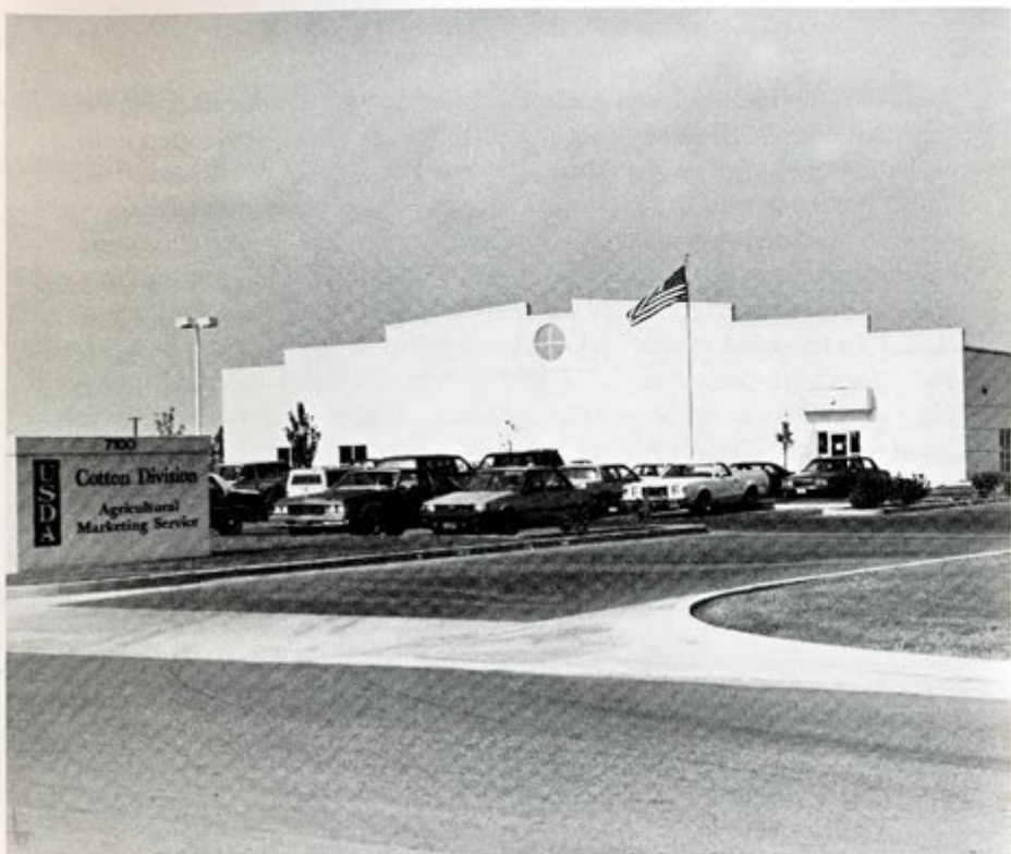
USDA operates 14 cotton classing facilities strategically located across the Cotton Belt. The facilities are specifically designed to use high-volume instrument (HVI) classification. Temperature and humidity inside the facilities are tightly controlled to ensure accurate and precise measurements of all samples.
