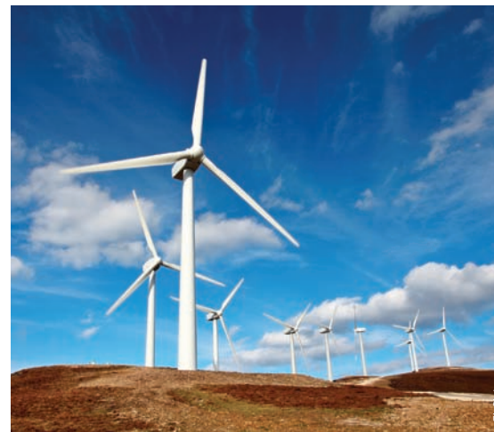
Modern Wind Farm
