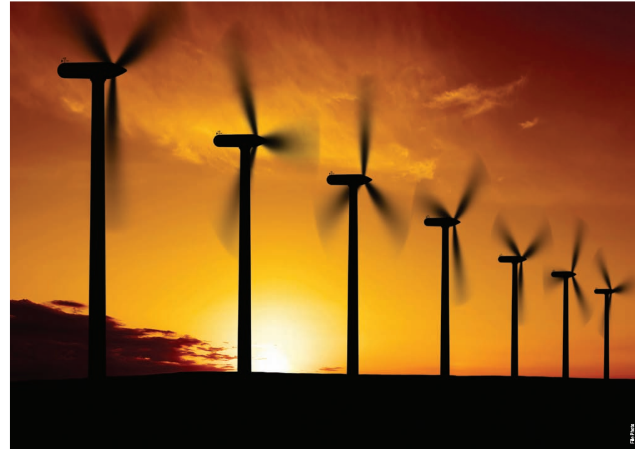
Modern Wind Farm
