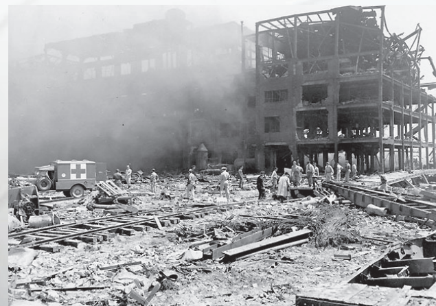
Destroyed Monsanto plant
