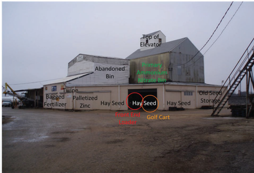
Storage of other combustible materials near fertilizer
