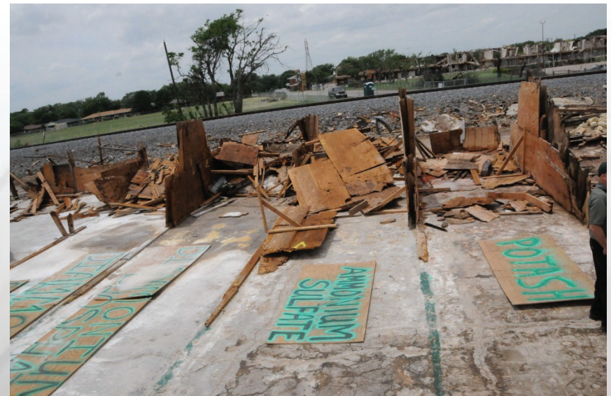
Facility and storage bins constructed of combustible materials
