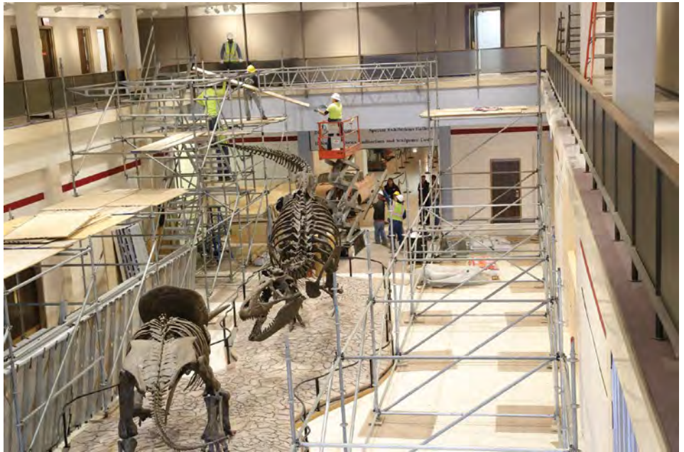
The museum under construction.
