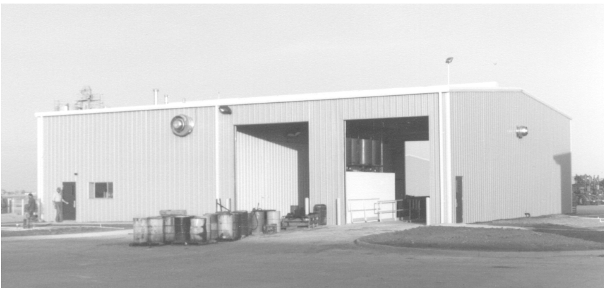
Figure 16. View looking northeast of the Tool building as rebuilt.
