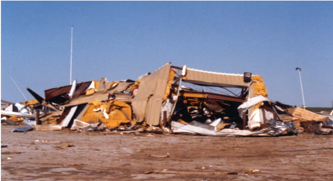
Figure 17. View looking east of the remains of the Shop building.
