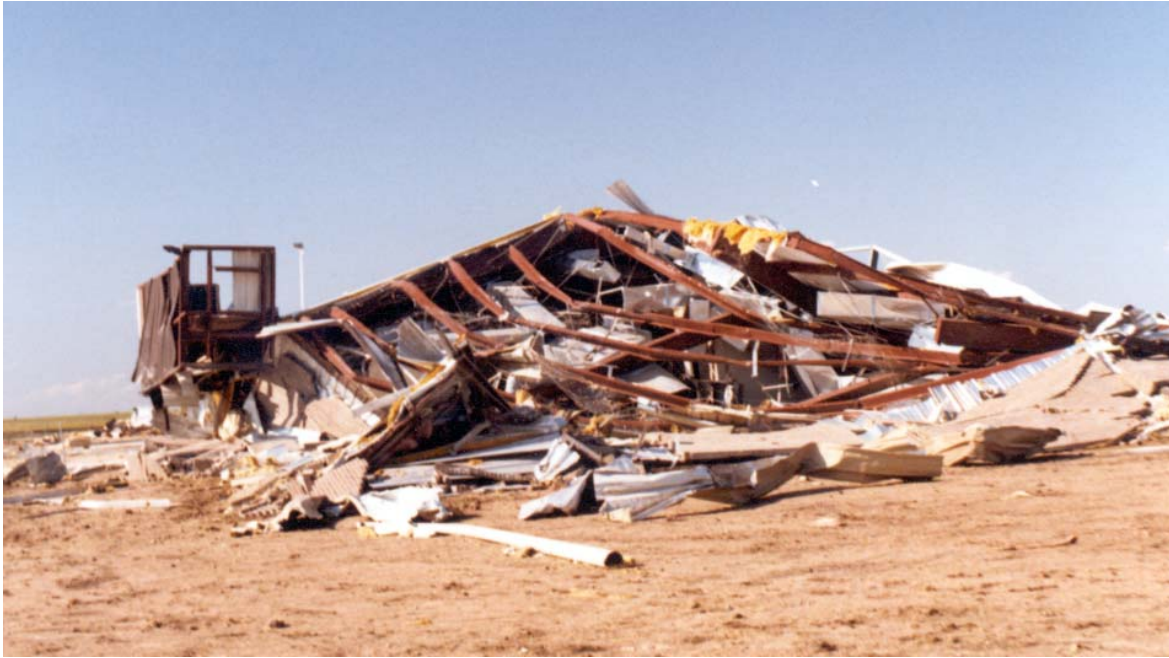
Figure 13. Damage to the Office building looking north. Note position of light standard.
