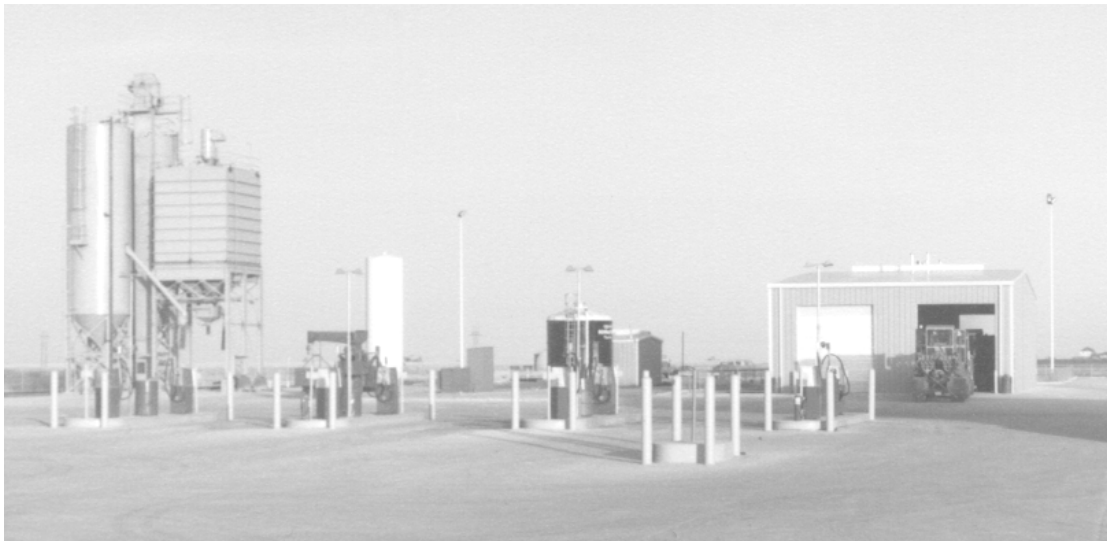
Figure 21. View looking west of Truck Wash building as rebuilt.
