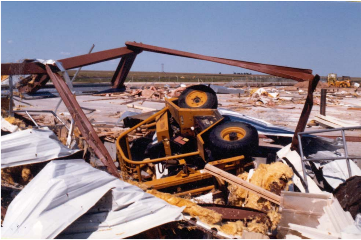
Figure 11. Remains of the Warehouse-Admixture building which was totally destroyed by the tornado
