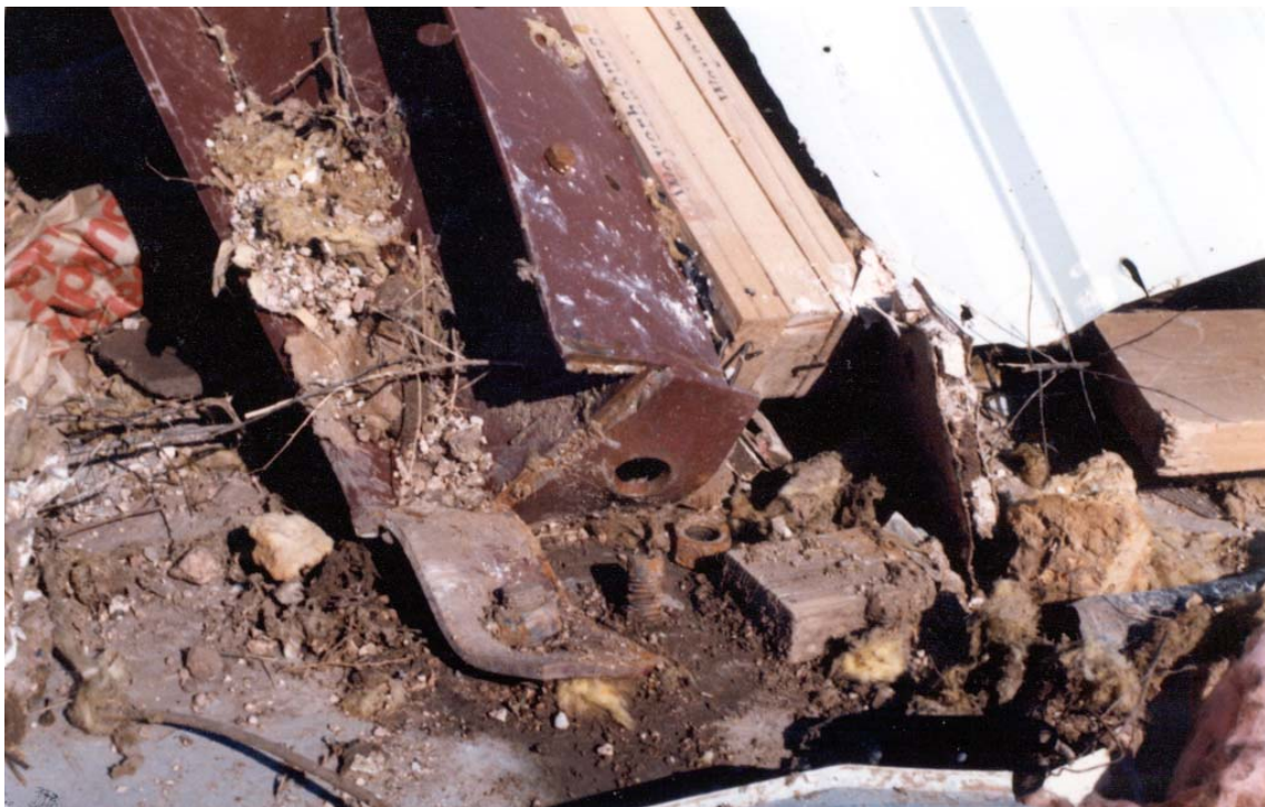
Figure 19. Example of column base plate tearing in the Shop building
