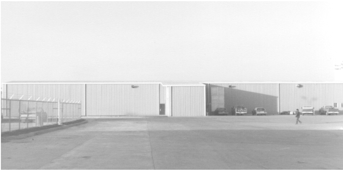
Figure 12. View looking north of Warehouse-Admixture building as rebuilt.
