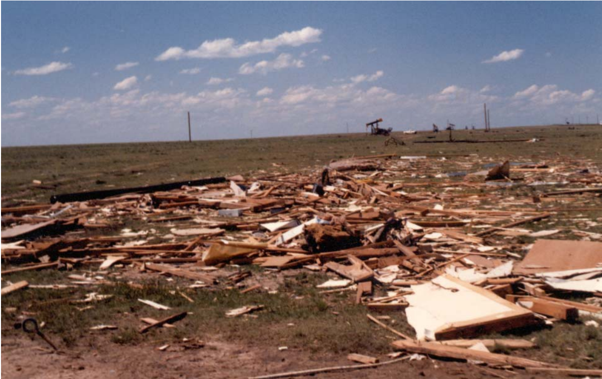
Figure 9. View looking north of the remains of a wooden building which was not anchored to its foundation.
