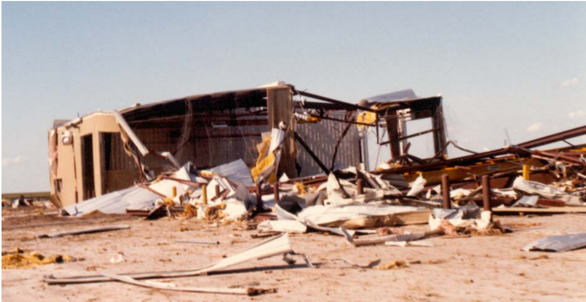
Figure 15. The Tool building was the largest building left standing after the tornado. View is looking north.
