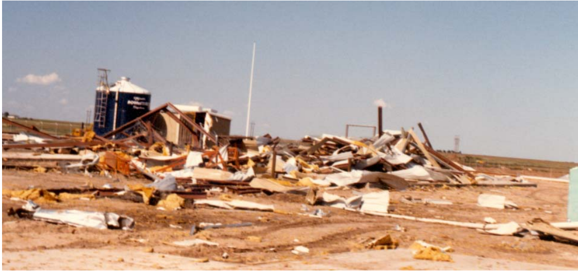
Figure 20. View looking east of damaged Truck Wash building.
