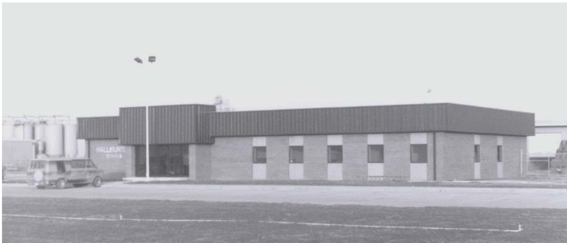
Figure 14. View looking northwest of the Office building as rebuilt.
