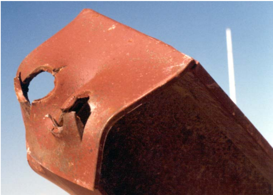
Figure 18. Example of column anchorage failure in the shop building. The anchor bolts pulled through the column base plate as the column was uplifted.
