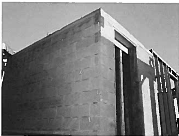
Above: An in-residence storm shelter under construction
