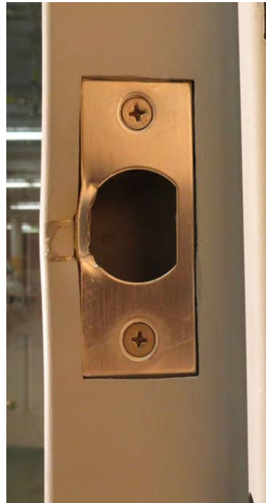
Figure 17: Deformed Deadbolt Strike.
