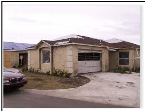
Figure 2: Negative pressure on OHD.
