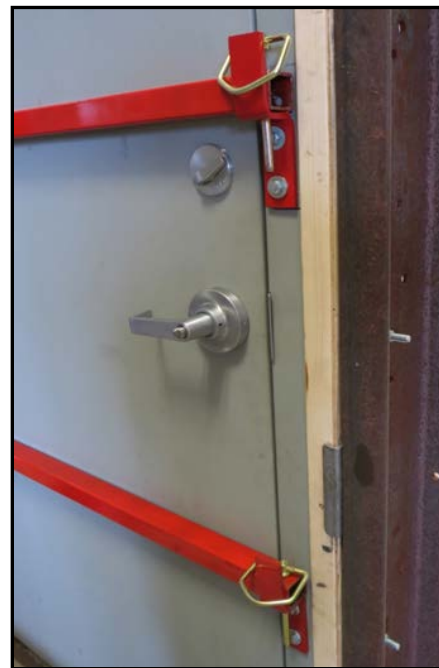
Figure 8: Shear Pins without Safety Pins 1 ½-in. x 1 ½-in. x 3/16-in. HSS
