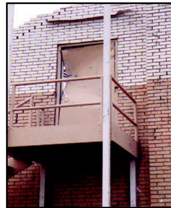
Figure 5: Exterior HM door impacted.
