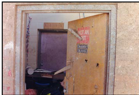
Figure 4: Multiple impacts on interior door.
