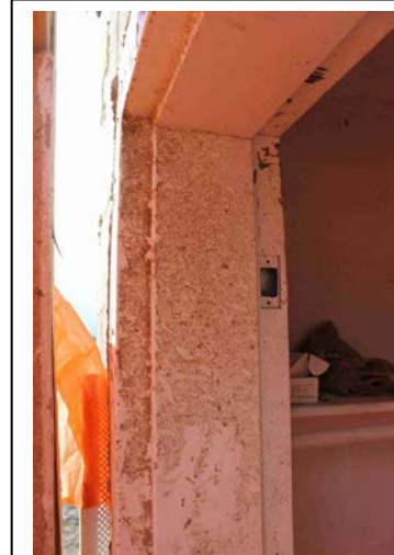
Door frame installed in shelter
