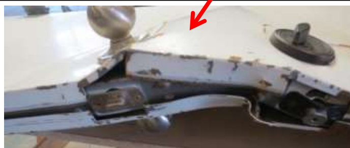
Door edge separation at latch and deadbolt location (door shown upside down to expose severe damage)
