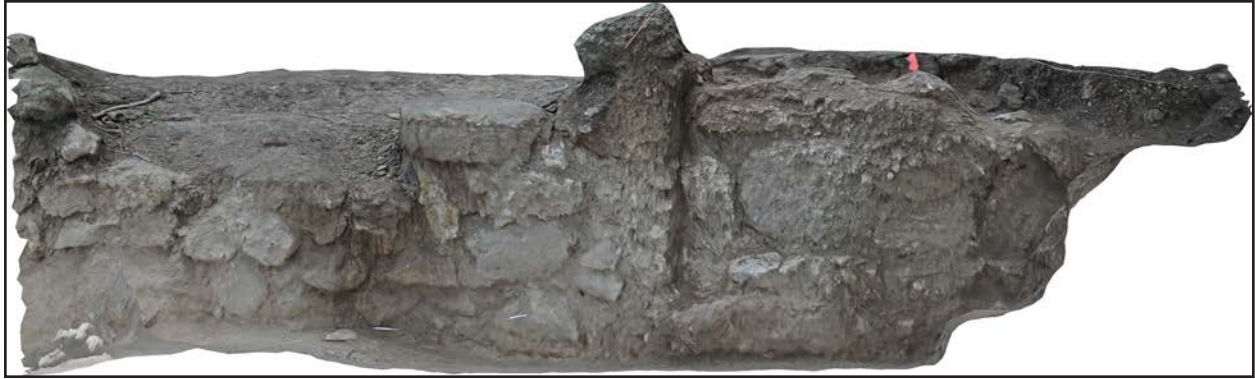
Figure 2.8. Orthophoto of southeast wall and infilled doorway jamb. View from west.
