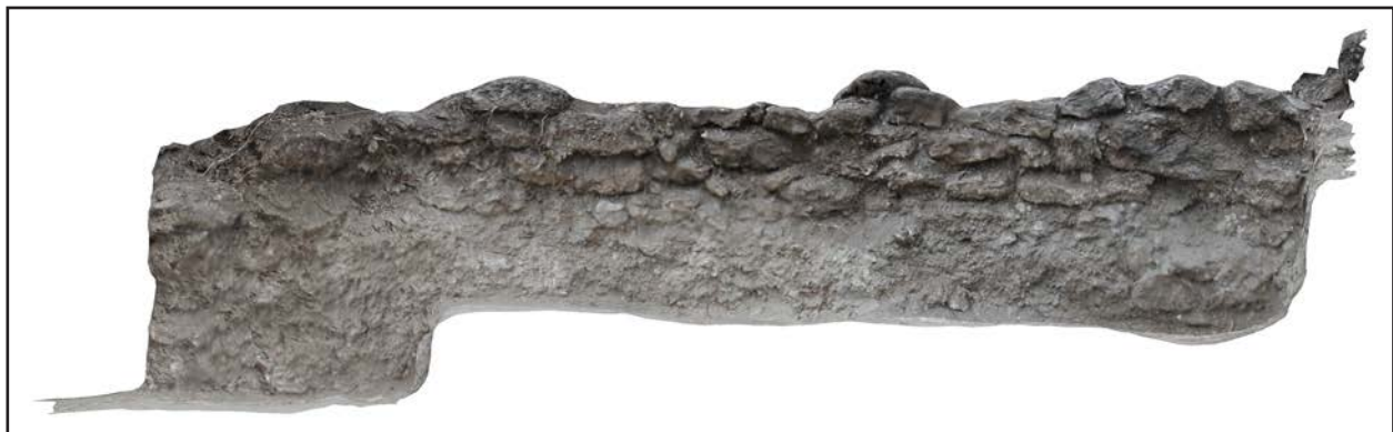
Figure 2.19. Orthophoto of Structure D-3, orientated north showing the northeast wall's two construction episodes.
