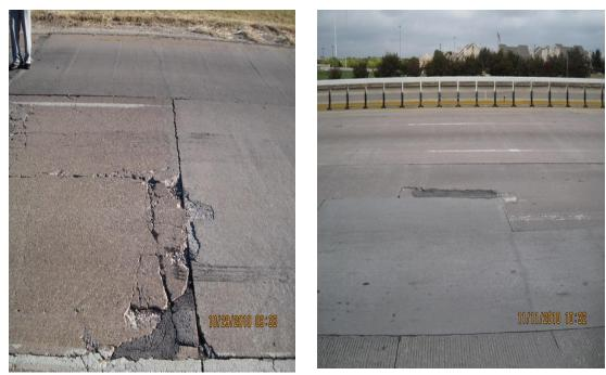
Figure 3-(a) Distress at repair jointFigure 3-(b) Distress at repair jointAbout 21 percent of the punchouts recorded in TxDOT PMIS occur at transverse
