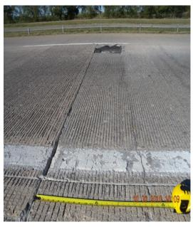
Figure 4-(a) Distress at transverse construction joint
