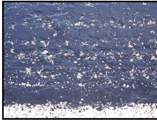
Figure 12. Freckling of prime coat binder on a dry base
