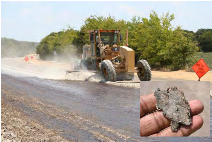
Figure 7 Application of worked-in (cut-in) prime on limestone base
