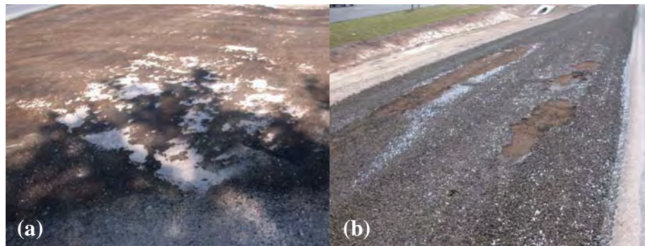
Figure 13 (a) Prime peeled-off at shaded area due to construction traffic (b) failed surface treatment due to construction traffic due to prime application when base is too wet.
