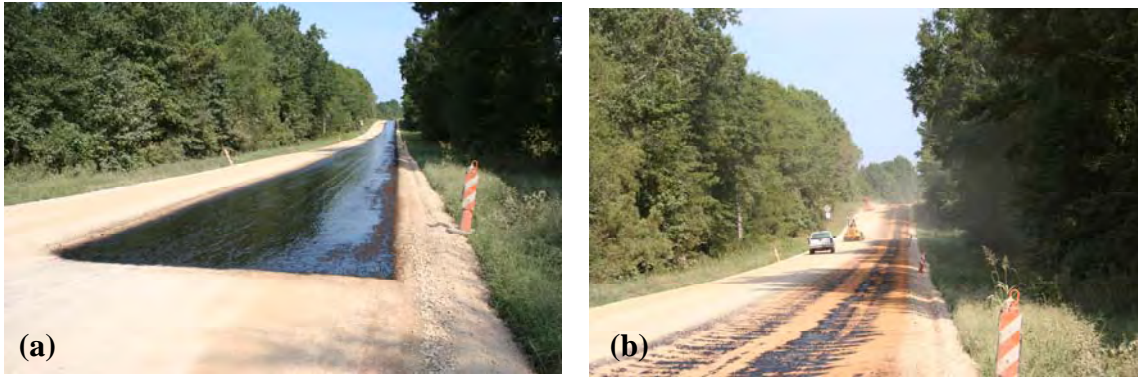
Figure 6. Spray Prime (a) MC-30 Cutback Prime (b) Blotting Sand Applied on Prime
