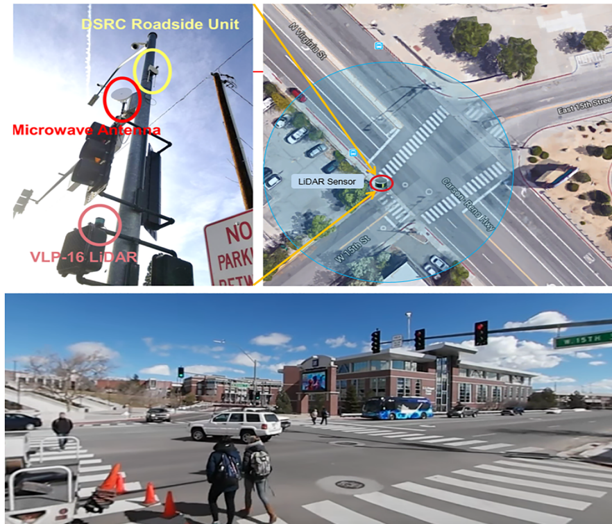
Fig. 1b. LiDAR sensor with other equipment and snapshot at one of the three intersections.
