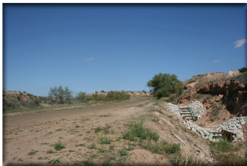
Before, During, & After EWP Project Top & Middle Photo Courtesy NRCS
