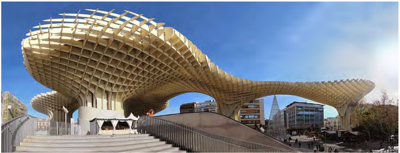
Metropol Parasol, Seville Spain - Jürgen Mayer
