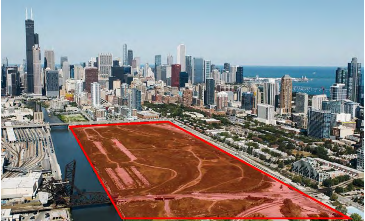
Figure: Project Site: "The 78" @ sloopin
