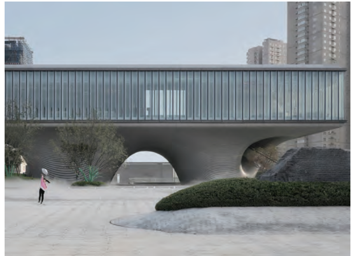
LAND Community Center, Xi'an, China, EID Architecture, 2020
