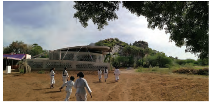
M.A.C. Community Center, Tiruvannamalai, India, Made in Earth, 2016
