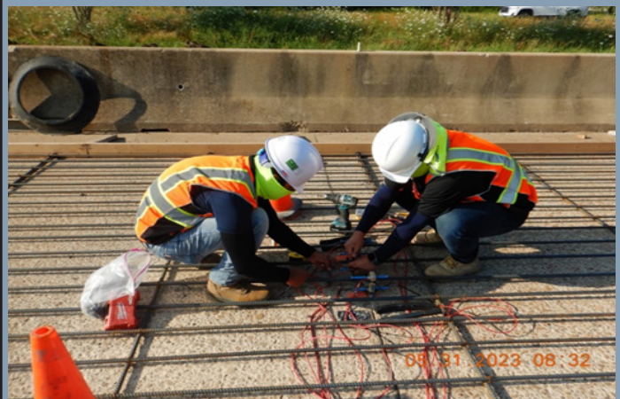
TechMRT researchers installing sensors
