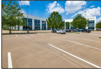
Eastern Parking Lot
