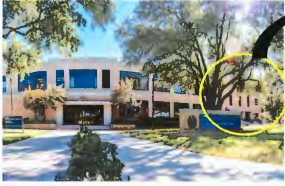
Sol Mayer Administration Building
