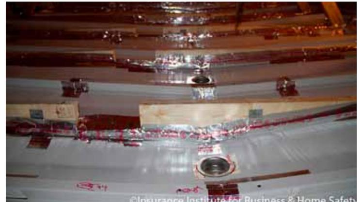
Figure 4. The drainage system installed in the attic of the duplex test house.
