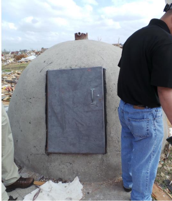
Figure 1.15. Dome shelter partially above-ground located in an EF-4 rated location (No. 40).
