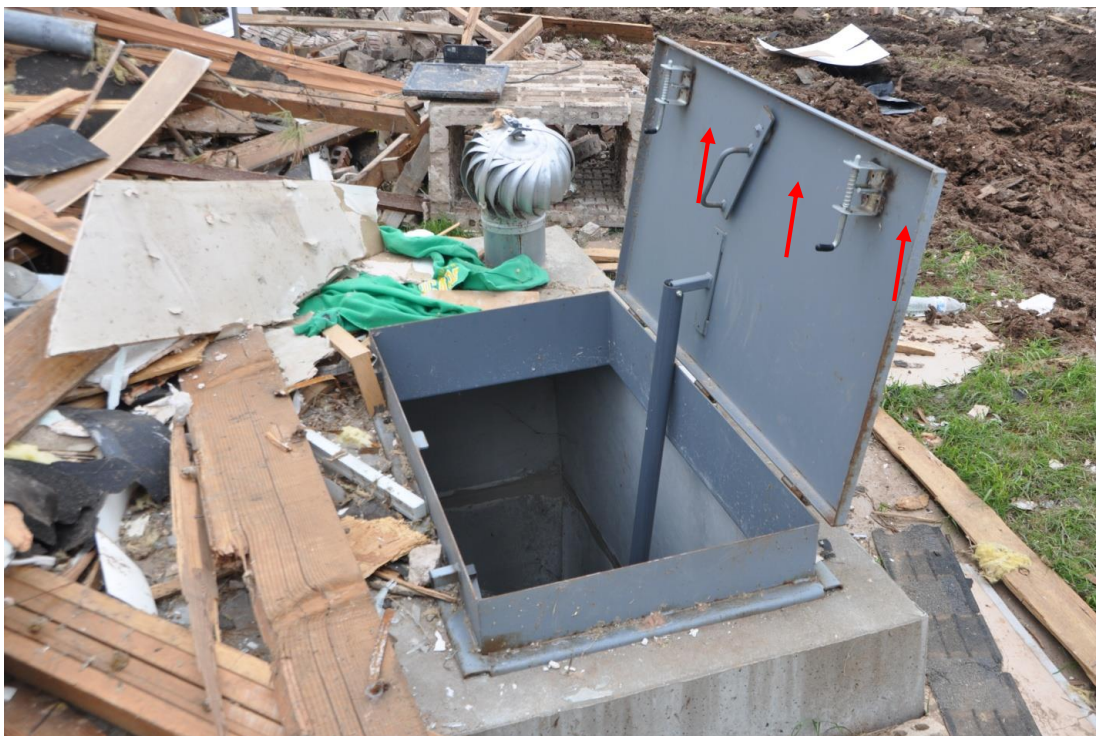
Figure 1.10. Flat top clam shell shelter with three locks at an EF-2 rated location (No. 17).
