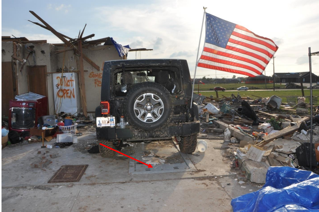
Figure 1.12. Tested shelter at a location assigned an EF-4 rating (No. 9). Car was present during the tornado.
