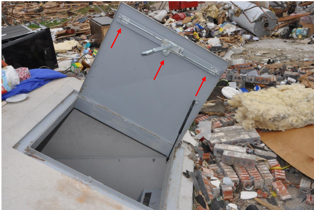
Figure 1.9. Clam shell shelter with a tested door that has three locks and three hinges at an EF-4 rated location (No. 28).
