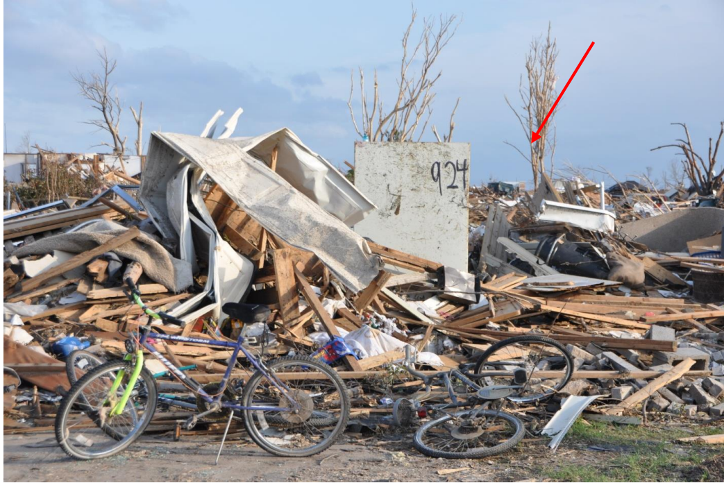
Figure 1.18. Above-ground tested steel shelter that performed very well in an EF-3 rated location (No 46).
