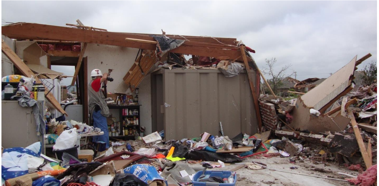
Figure 1.16. An above-ground tested shelter that survived EF-4 wind speeds (No. 25).
