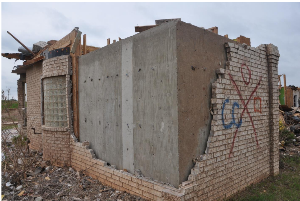
Figure 1.17. An above-ground, concrete shelter that also served as a walk-in closet at an EF-2 rated location (No. 49). The concrete was tested, but the door was not.
