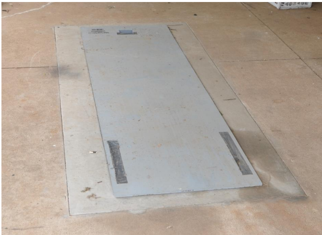
Figure 1.13. Tested NSSA shelter at a location assigned with an EF-0 rating (No. 61).
