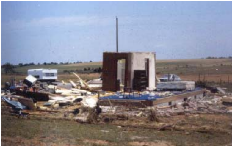
Figure 2. Farm house destroyed by the tornado. Interior walls remain standing around bathroom. Damage to this house was rated F-3 on the Fujita scale.
