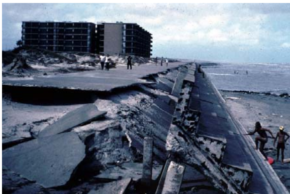
Figure 5. Seawall on North Padre Island was severely damaged by wave action during Hurricane Allen.
