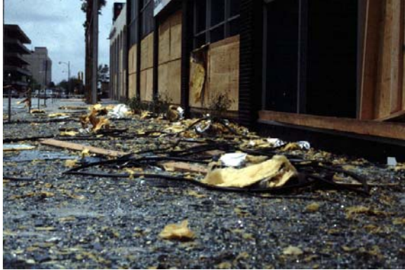
Figure 3. Window glass debris at base of Guaranty Bank Building.
