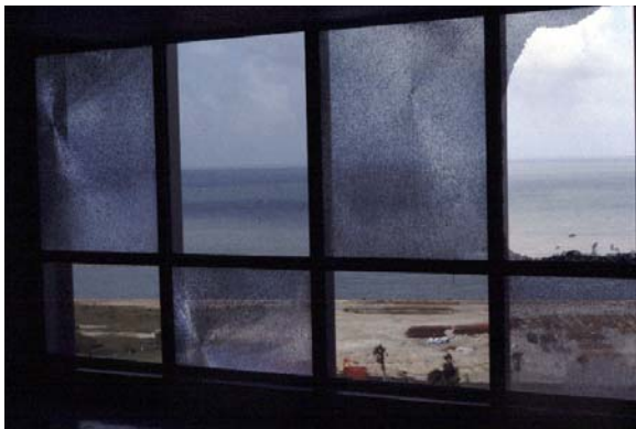
Figure 4. Tempered insulating glass failures from roof gravel impact at Spohn Hospital.
