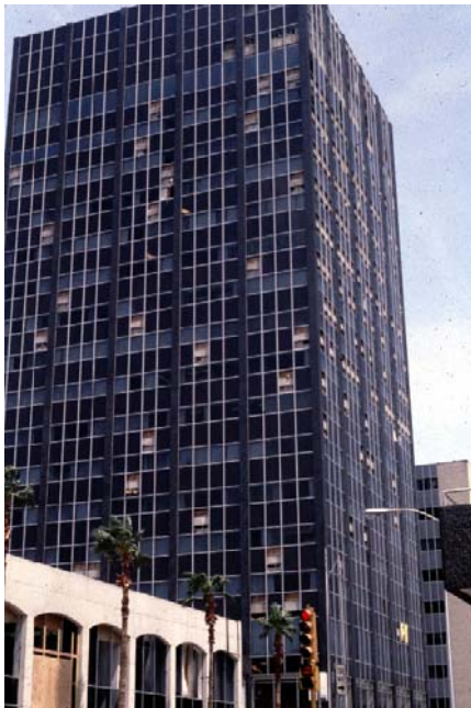
Figure 2. Many windows were lost at the Guaranty Bank Building during Hurricane Allen.
