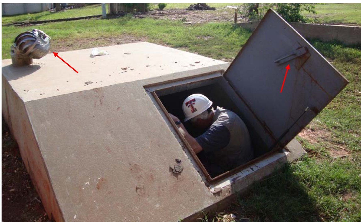
Figure 8. Clam shell shelter with an insufficient locking system and damaged vent at an EF-2 rated location (No. 3).
