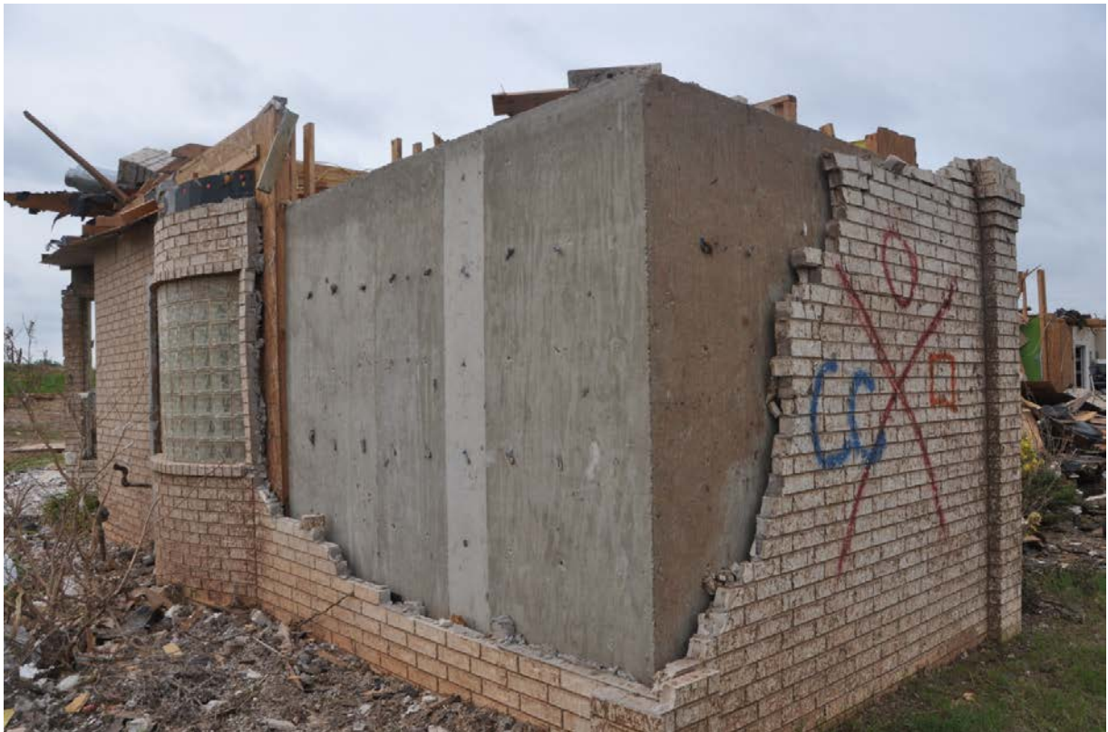
Figure 17. An above-ground, concrete safe room that also served as a walk-in closet at an EF-2 rated location (No. 49). The concrete was tested, but the door was not.
