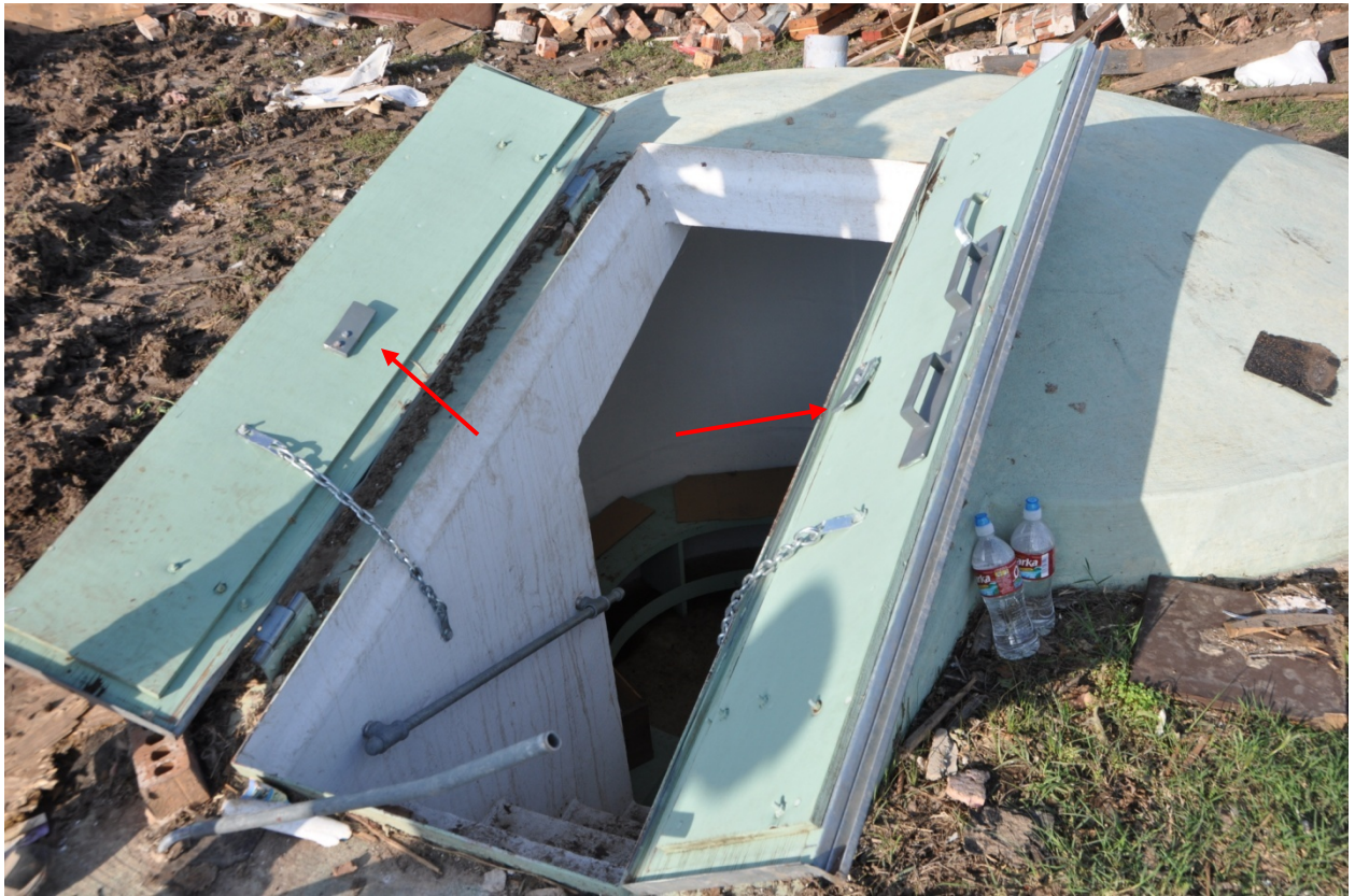
Figure 14. Dome shelter with an inadequate door system that included a plywood and light gage sheet metal clad door, single locking point, and ventilator removed at an EF-3 rated location (No. 43).
