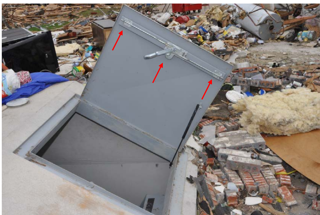
Figure 9. Clam shell shelter with a tested door that has three locks and three hinges at an EF-4 rated location (No. 28).
