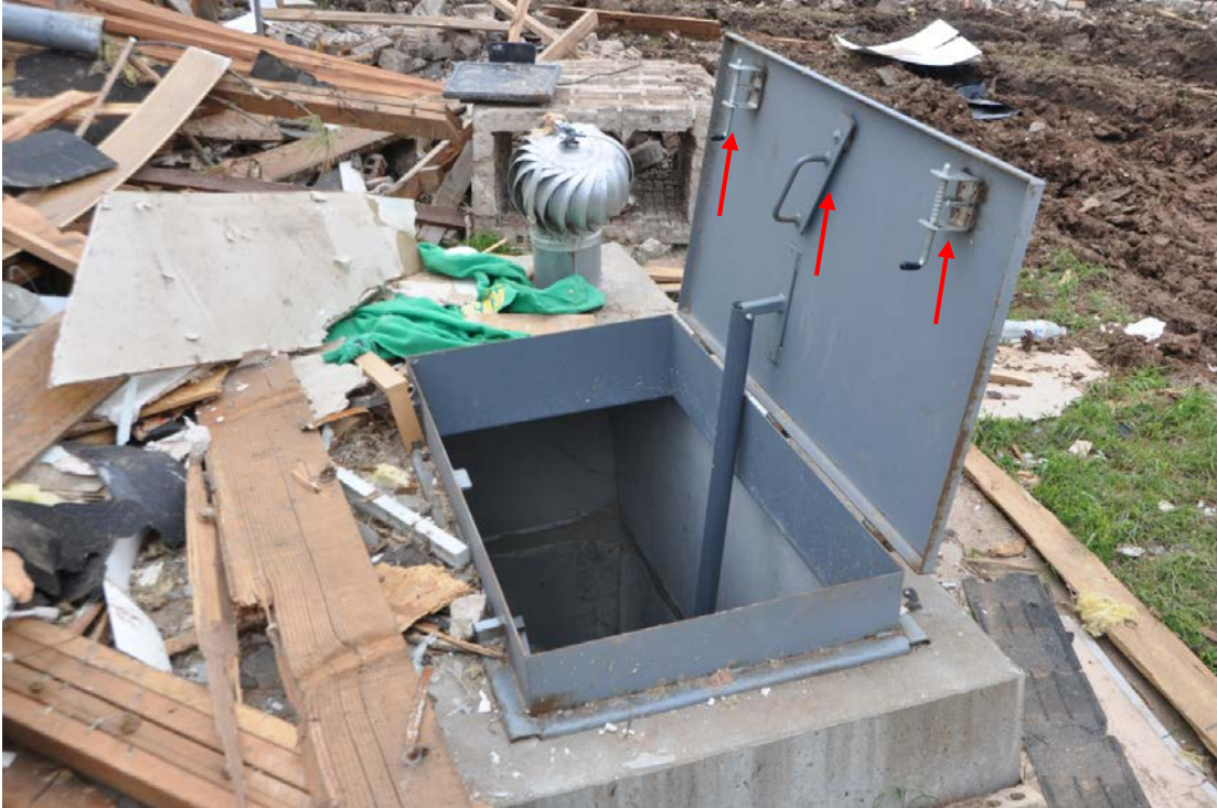
Figure 10. Flat top clam shell shelter with three locks at an EF-2 rated location (No. 17).
