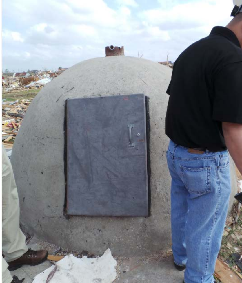
Figure 15. Dome shelter partially above-ground located in an EF-4 rated location (No. 40).
