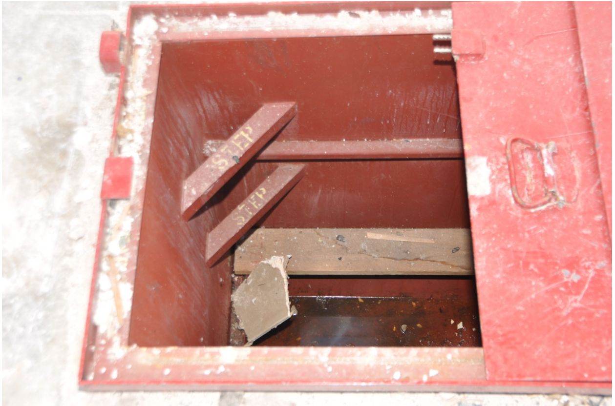
Figure 11. In-garage storm shelter with inadequate stairs, locking system, and flooding in the bottom at an EF-3 rated location (No. 12).
