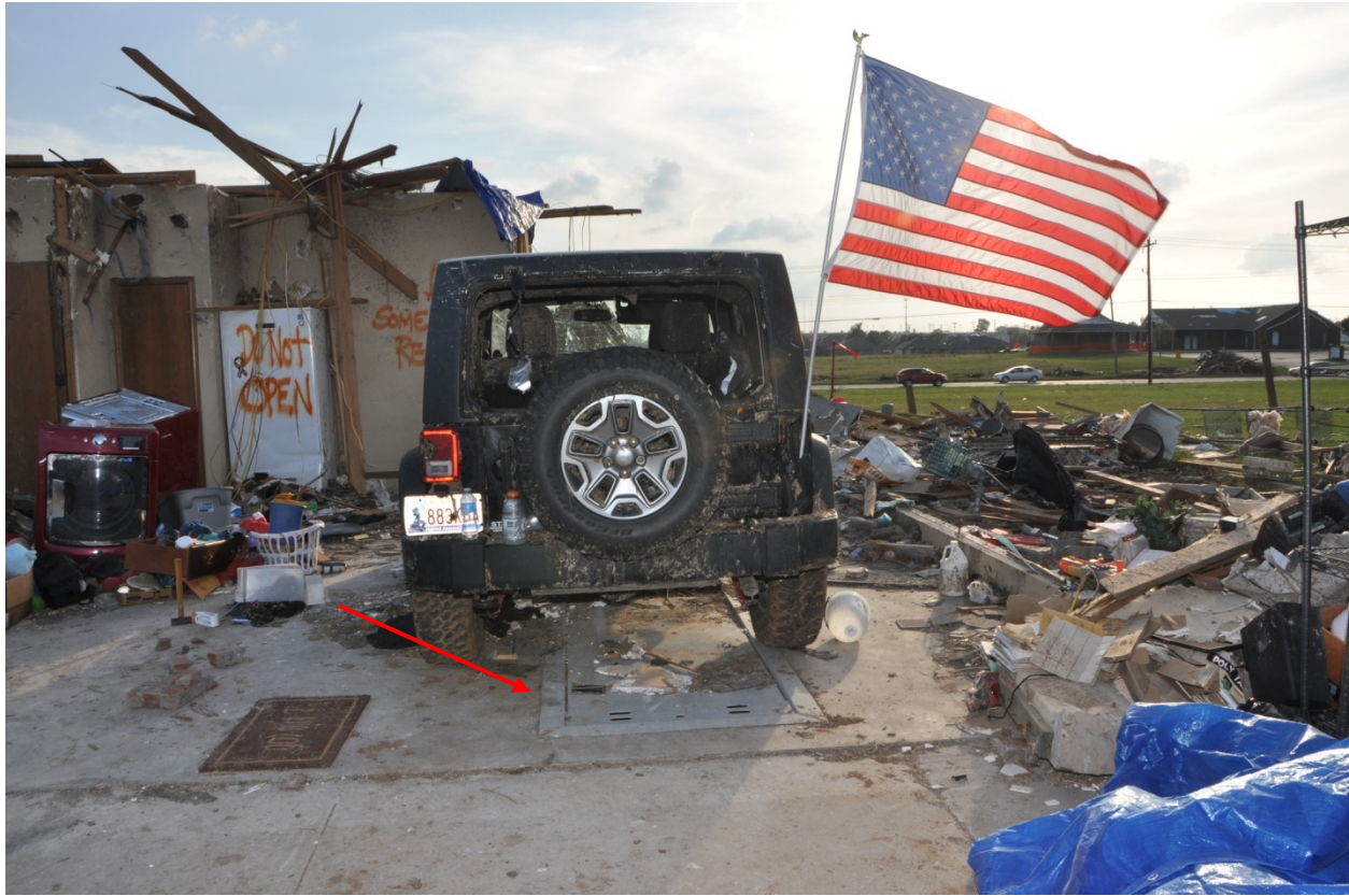
Figure 12. Tested shelter at a location assigned an EF-4 rating (No. 9).
