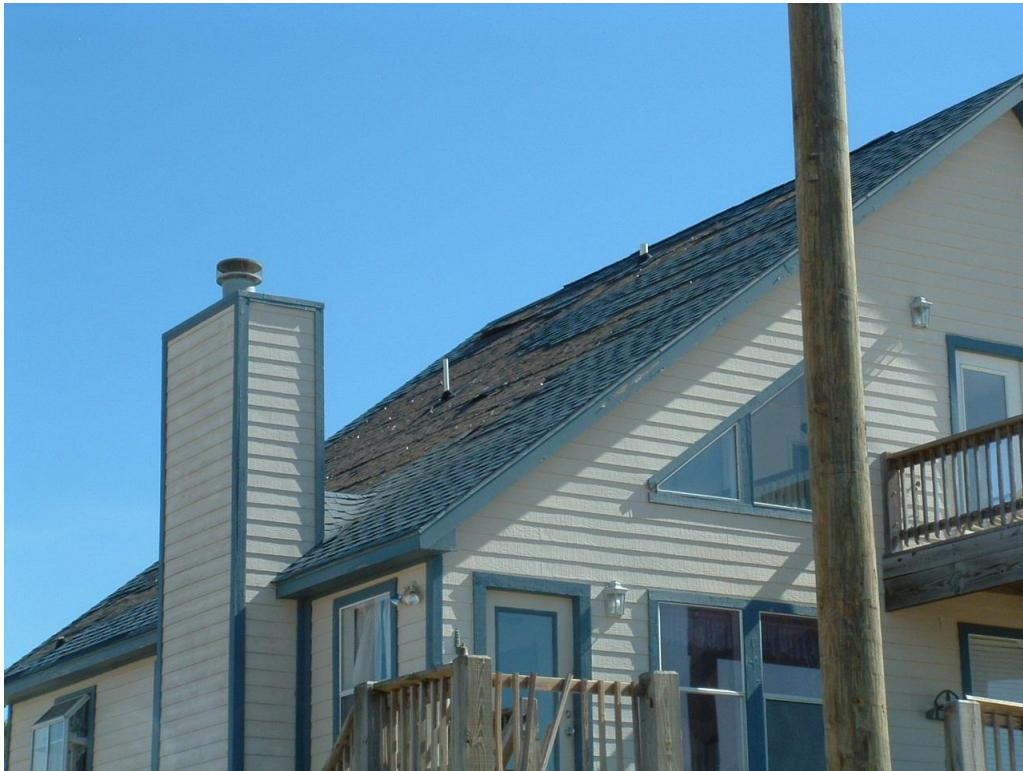
Figure 1 Roof damage from Hurricane Ike
