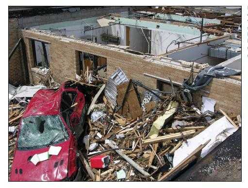
Figure B8-10. Representative quantity, size, and type of debris that is often generated by a strong or violent tornado. The building damage at this site was indicative of an EF3 tornado. (Greensburg, KS, 2007)
