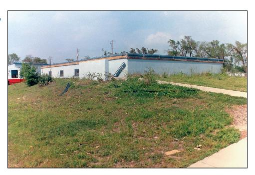
Figure B3-11. Soil cover over a safe room relieving the requirement for debris impact-resistance
