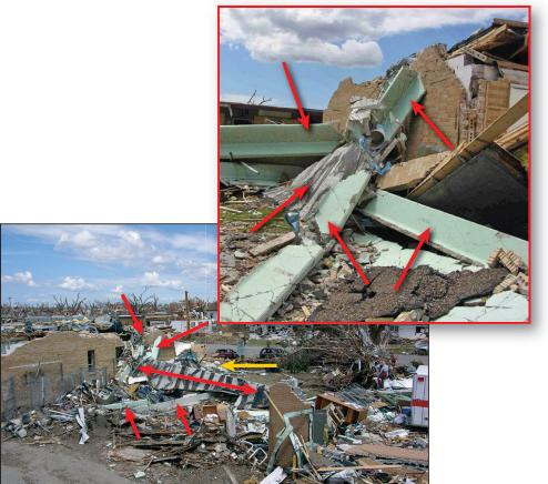
Figure B8-6. Large debris: Roof precast twin tees (red arrows) blew off a hospital and struck another portion of the building (see inset; yellow arrow shows direction of view). One of these flew approximately 80 feet. The building damage at this site was indicative of an EF3 tornado. (Greensburg, KS, 2007 tornado)
