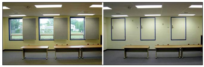
Figure A4-5. Interior operated safe room shutters in multi-purpose classroom/safe room. Image on left is normal usage; image on right shows shutters in 'lock down' position where they are closed and latched
