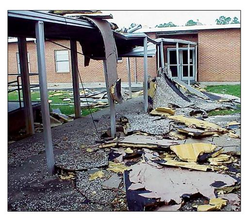
Figure B8-2. Medium debris: Pieces of a built-up roof from Hurricane Katrina (MS, 2005)
