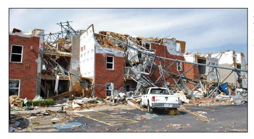
Figure B3-12. Lay down hazard: failure of a large communications tower onto a building (Joplin, MO, 2011 tornado)
