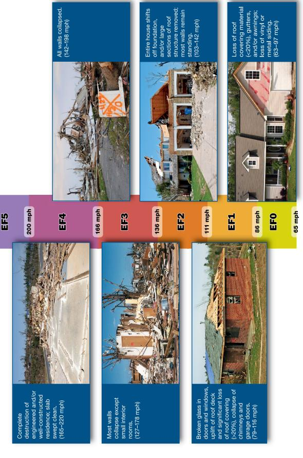
Figure A2-1. Typical tornado damage descriptions to one- and two-family dwellings and their corresponding intensity according to the EF Scale (wind speeds are estimated 3-second-gust wind speeds)
