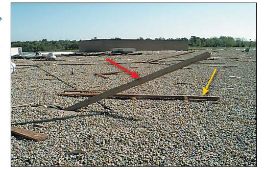
Figure B8-4. Large debris: Steel beam that blew into a school (Greensburg, KS, 2007 tornado)
