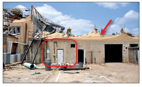
Figure B3-14. Collapse hazard: the story above an Emergency Operations Center collapsed. Masonry walls (red arrow) and part of the roof structure fell onto the second story floor slab above the EOC (Tuscaloosa, AL, 2011 tornado) (SOURCE: FEMA P-908, RECOVERY ADVISORY 6)
