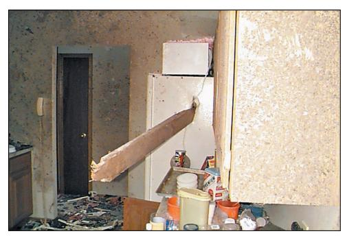
Figure B8-11. Refrigerator pierced by a 2x6. The portion of the 2x6 that is visible was 4 feet 8 inches long. It went several inches into the freezer compartment.
