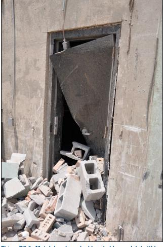
Figure B8-1. Metal door breached by wind-borne debris (this door was not designed to resist debris). (Tuscaloosa, AL, 2011 tornado)
