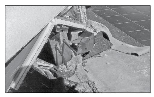
Figure B3-9. Two steel columns failed at their connection to the foundation when the anchor bolts that secured the column released from the concrete (embedment failure) while the anchor bolts that secured the column on the right experienced a ductile failure
