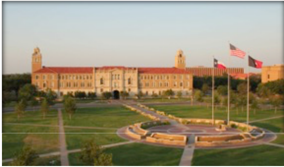
Figure 15: TTU Administration Building
