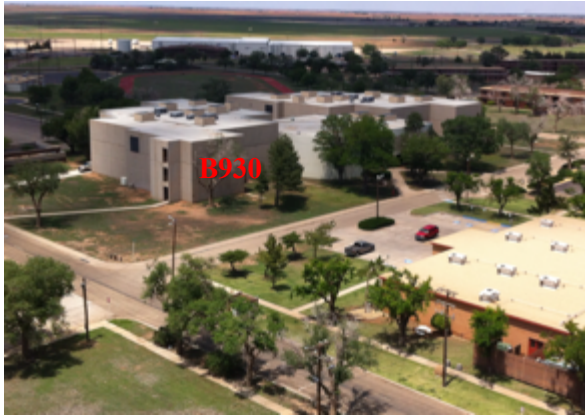
Figure 19: Former Flight Simulator Building
