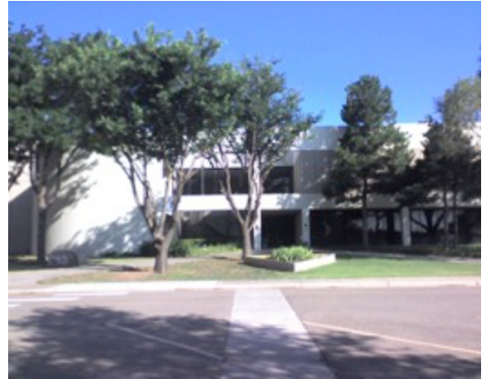
Figure 20: B930 Walkway to Parking
