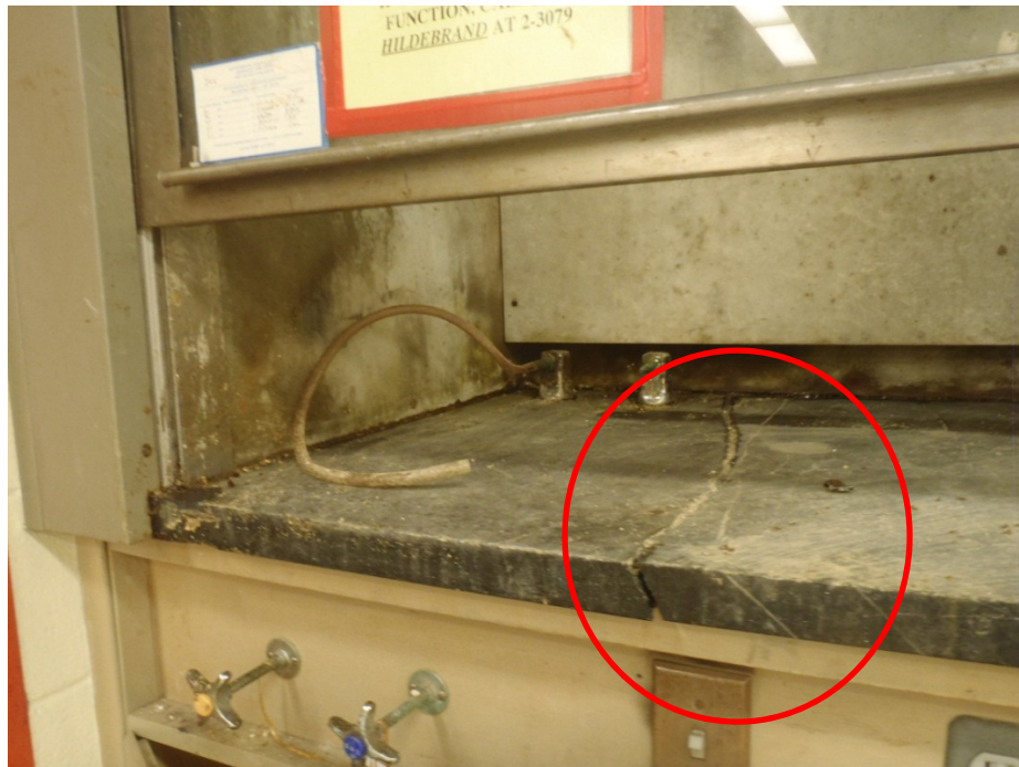
Image 1. Area where incident occurred. Prominent crack in fume hood countertop.
