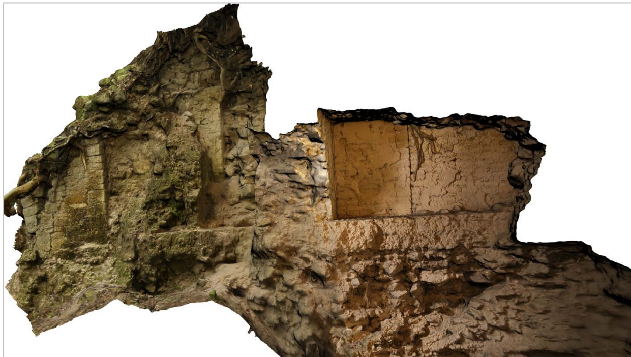
Figure 2. SfM orthophoto, view to the south, of the interior of the uppermost trench and tunnel on the eastern side of Structure A-15 showing various architectural features, after Willis et al. (2014:Figure 2.7). The room exposed in the tunnel (upper right in image) is not accessible and had never been documented before.
