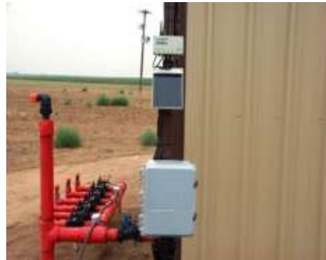
Valve bank with air relief
