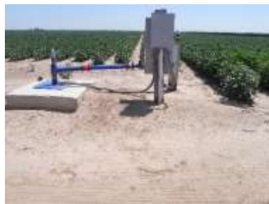
Well pad for irrigation
