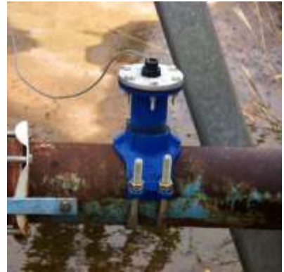
Electronic flow meter
