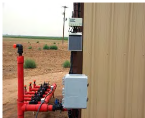
Valve bank with air relief
