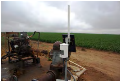
Surface turbine irrigation well
