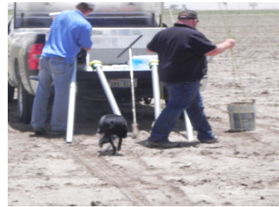
Moisture probe installation
