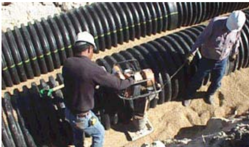
Figure 1. HDPE Pipe Installation on US-83, San Angelo
