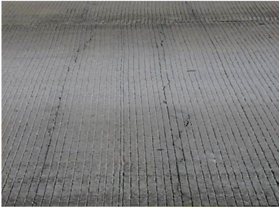
FIGURE 6 Typical CRCP section with 100 % recycled aggregates.
