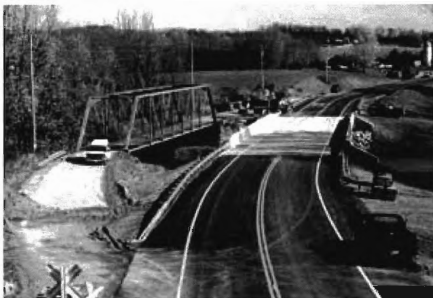
Figure 4.1 Use of a Temporary By-pass Bridge during Bridge Reconstruction
