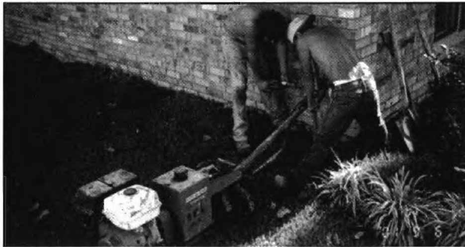
Figure 5.2 3-foot-wide, 3-foot-high Specialty Rig Drills Holes up to 18-inch Diameter and 20-foot Depth (Source: S & W Foundation, Richardson, Texas)
