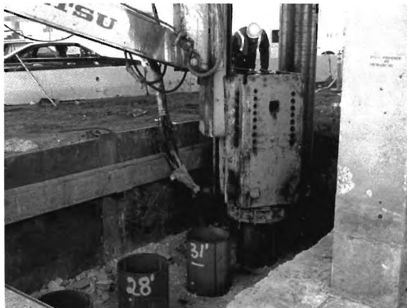
Figure 5.7 Installation of Additional Piles around Old Pile Cap (Source: bbuckland@mandelpipe.com )
