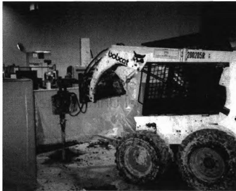
Figure 5.3 5-foot 6-inch-wide, 6-foot 9-inch-high Specialty Rig Drills Holes up to 60-inch Diameter and 75-foot Depth (Source: S & W Foundation, Richardson, Texas)
