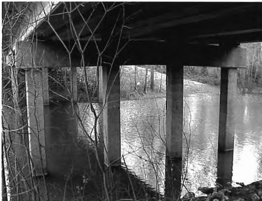
Figure 5.13 Off-system Bridge on County Road 569 at Oyster Creek
