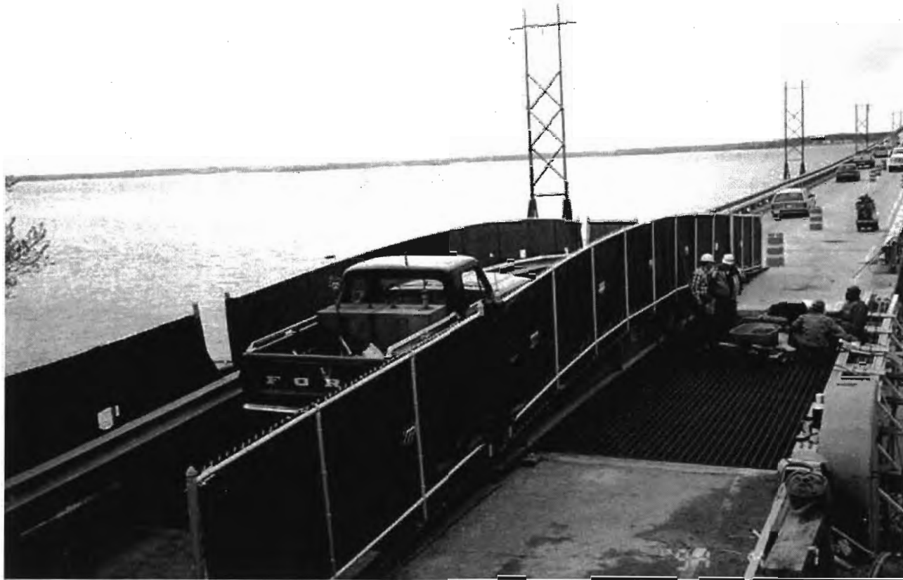
Figure 5.11 Temporary Bridge in Use During Bridge Reconstruction
