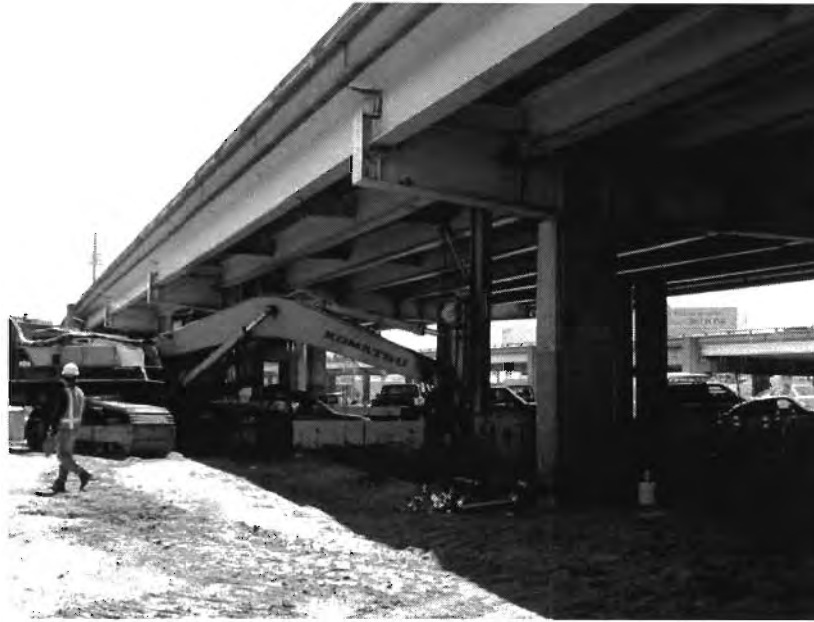
Figure 5.6 Use of Limited Headroom Pile Driver in the Retrofit of Pier Foundations in the San Francisco-Oakland Bay Bridge (Source: bbuckland@mandelpipe.com )
