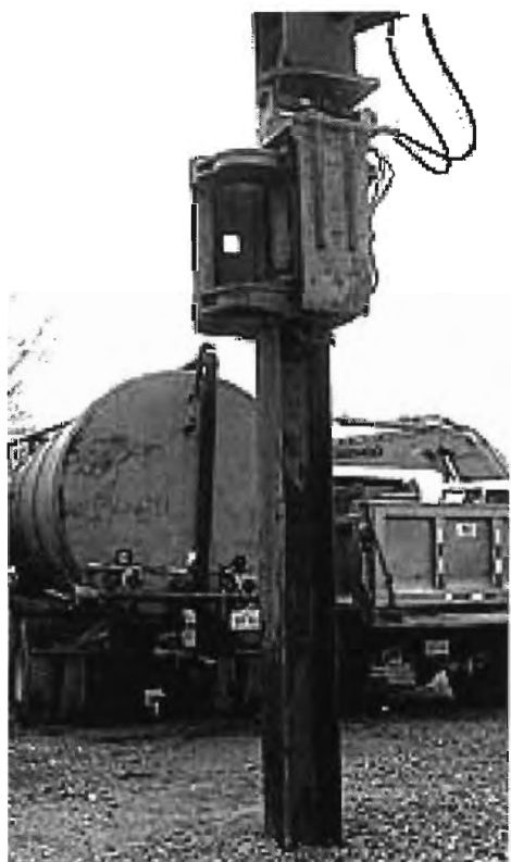
Figure 5.5 Robotic Vibratory Pile Driver Attached to an Excavator
