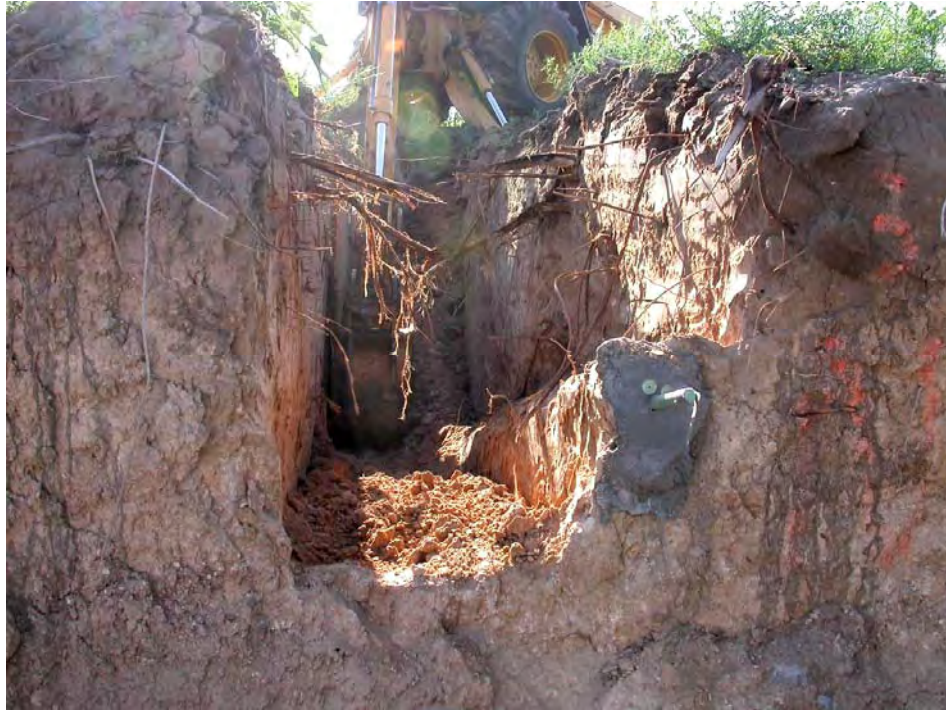
Figure 5.25 Remove Soil from the Sides of Nails
