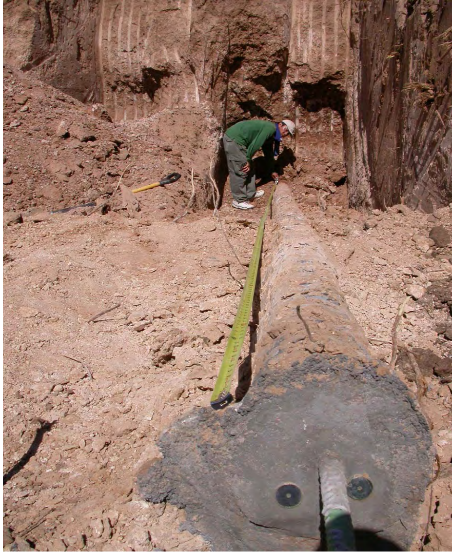
Figure 5.28 Measuring and Recording Actual Nail Grout Condition
