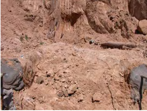
Exposed Nail #27 (left) joined with Nail #28 at 18'4" and grout ends at 27'
