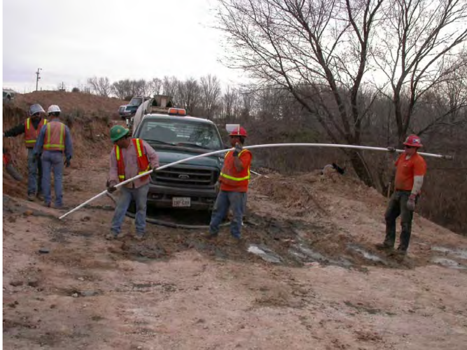
Figure 4.36 The 20 feet long PVC Tremie Pipe Used in Phase 2
