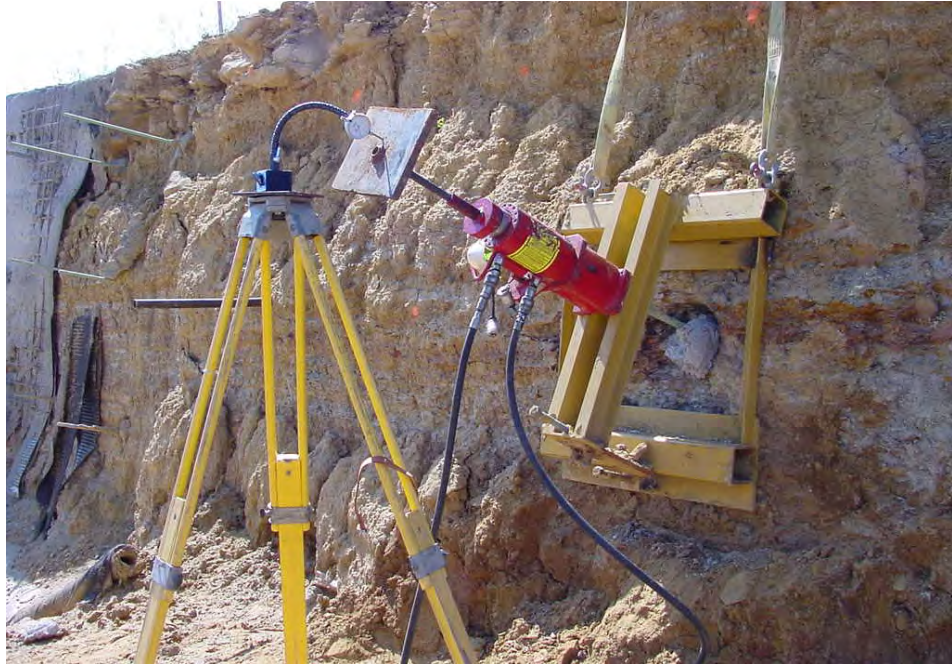
Figure 2.7 Test Setup Used for Soil Nail Load Testing
