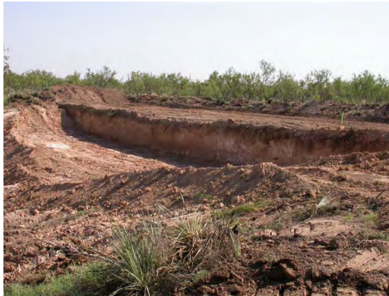
Figure 4.15 View of the Construction Site after Completion of the Excavation
