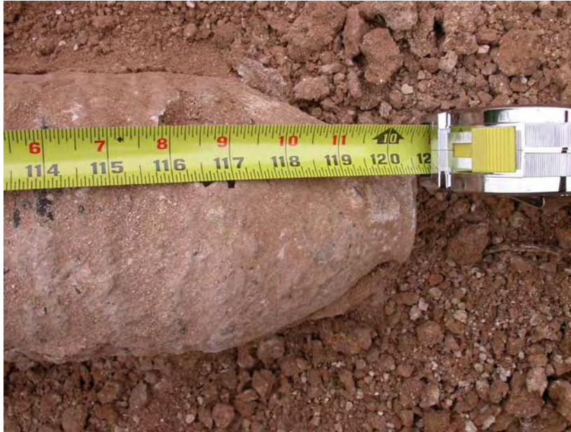
Figure 5.51 Nail No.5 Grout Column Ends at 10ft
