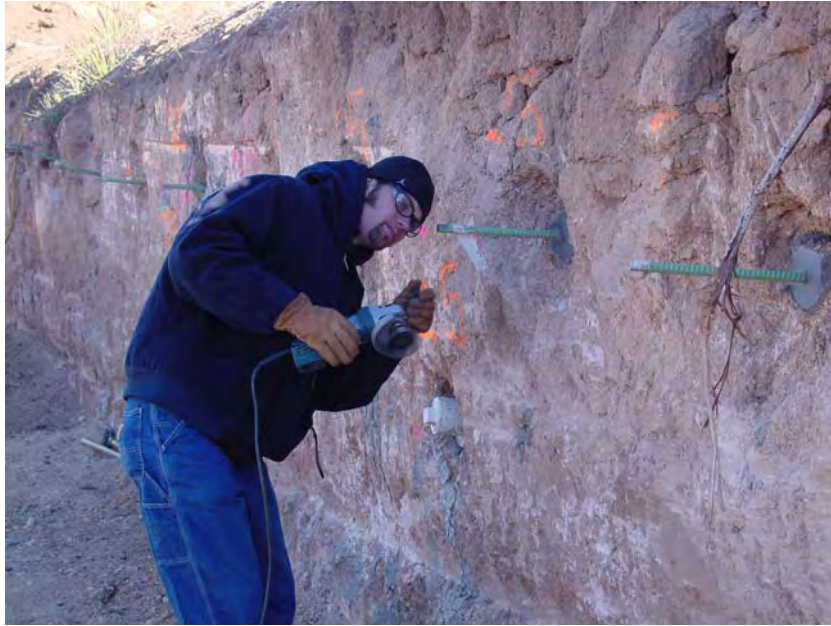
Figure 5.21 Grinding the Steel Tendon to Achieve Electrical Contact
