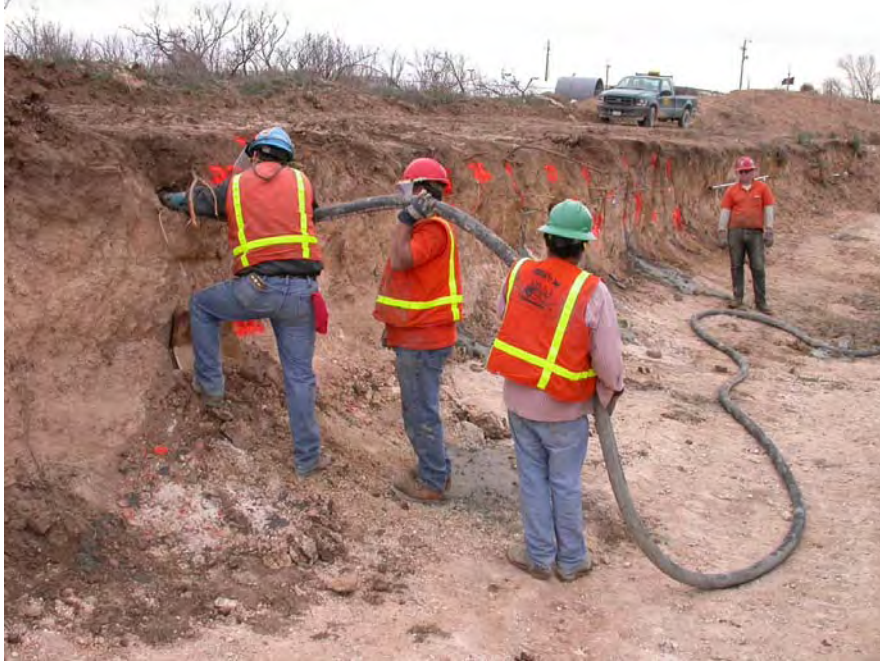
Figure 4.34 Grouting Drillholes before Inserting Steel Tendons
