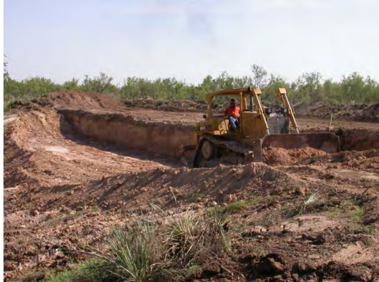
Figure 4.14 Site Cleaning and Soil Excavation
