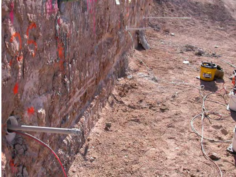
Figure 5.16 Three Boreholes Embedded with PVC Pipes
