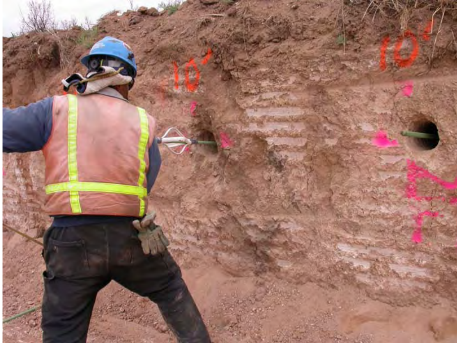
Figure 4.18 Insertion of Steel Tendons into Drillholes
