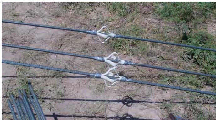
Figure 6.5 – Common #6 Rebar with Centralizers
