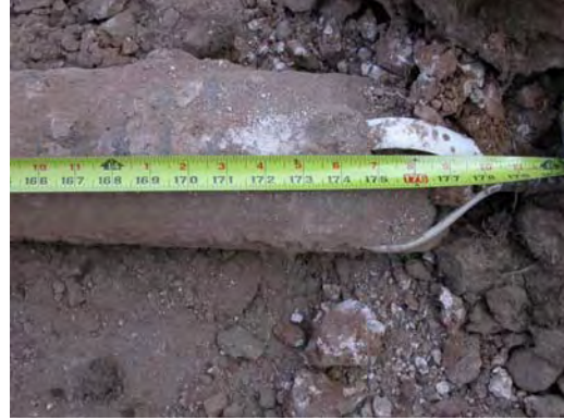
Grout ends at 14'8"
