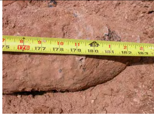
Grout passes through the middle foam, ends at 15'2"
