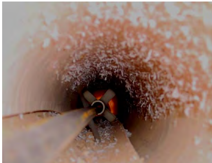
Figure 6.3 – Inside of the PVC Tube with Tendon and Centralizers in Place
