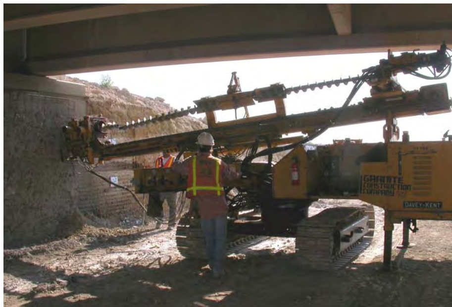
Figure 2.4 Drilling Hole for Soil Nail Installation
