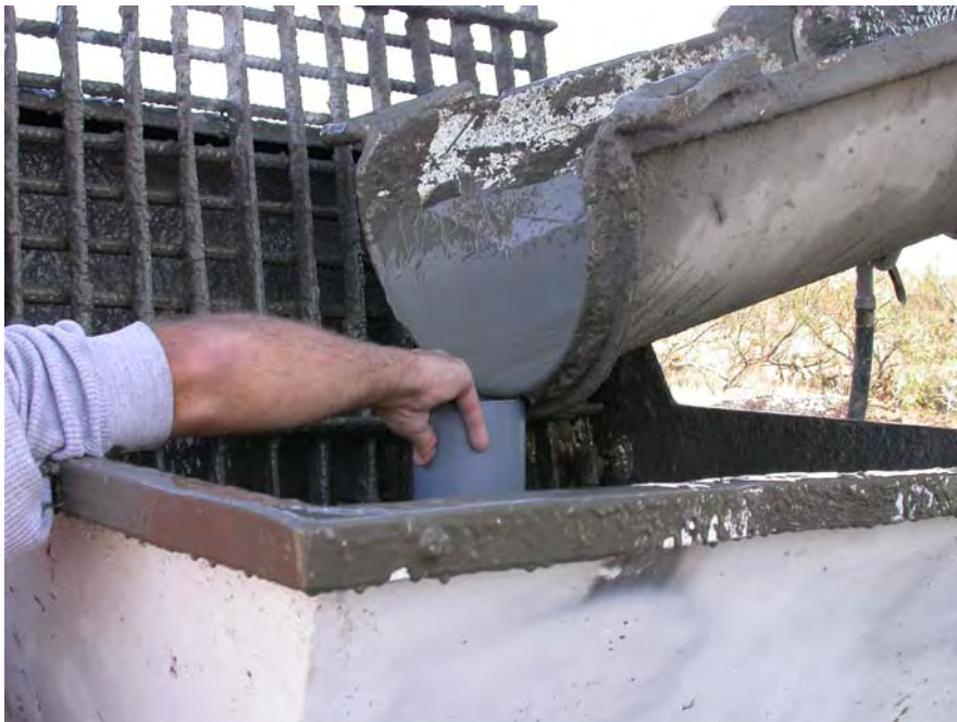
Figure 4.21 Sampling Grout for Testing
