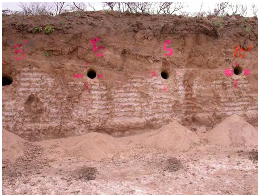
Figure 4.17 View of the Wall Face with Drillholes
