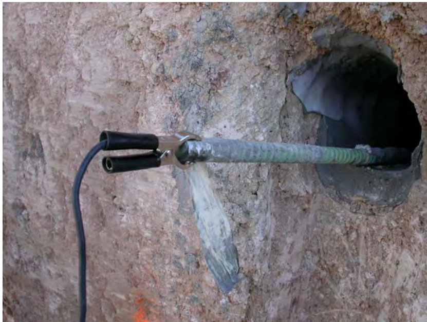
Figure 5.22 Attaching Cable on Steel Tendon
