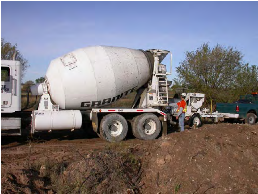
Figure 4.20 Grouting Truck and Grout Pump
