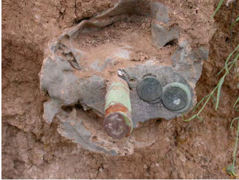
Figure 5.12 Epoxy Glue was Used to Glue the Washer with the Grout
