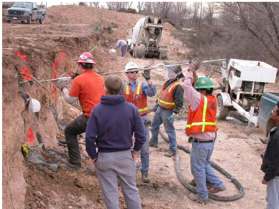
Figure 4.35 Inserting Steel Tendons after Partial Grouting of the Hole
