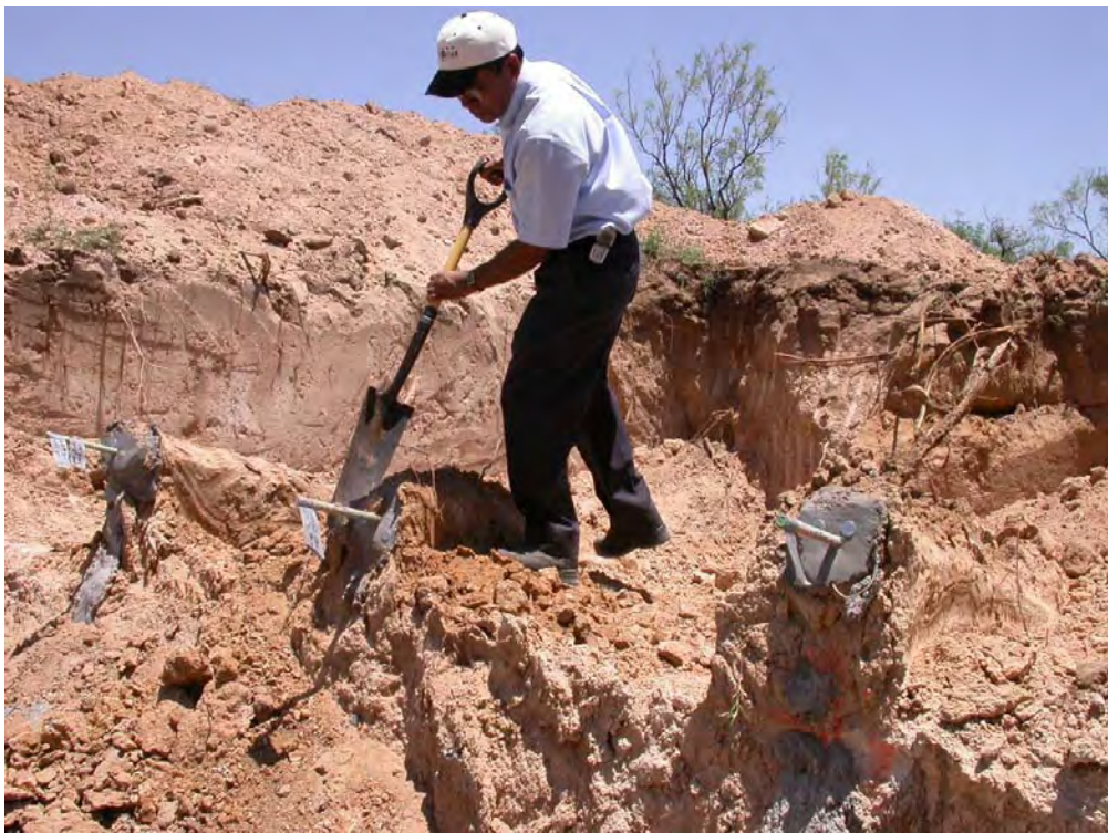
Figure 5.27 Using Hand Shovel for Final Cleanup
