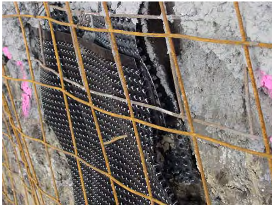
Figure 2.6 Use of Prefabricated Vertical Geocomposite Drainage Strips
