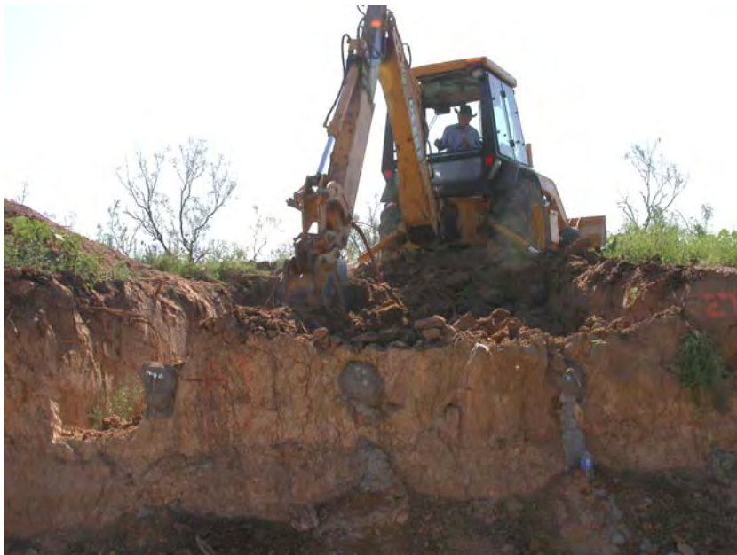
Figure 5.24 Remove Soil from the Top of Nails
