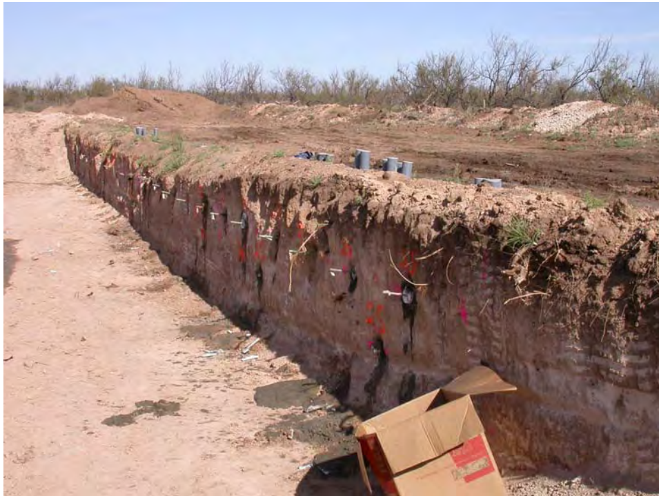
Figure 4.27 Completed Test Soil Nail Wall
