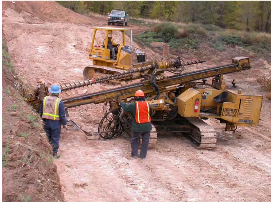
Figure 4.16 Drilling Holes for Installation of Test Soil Nails
