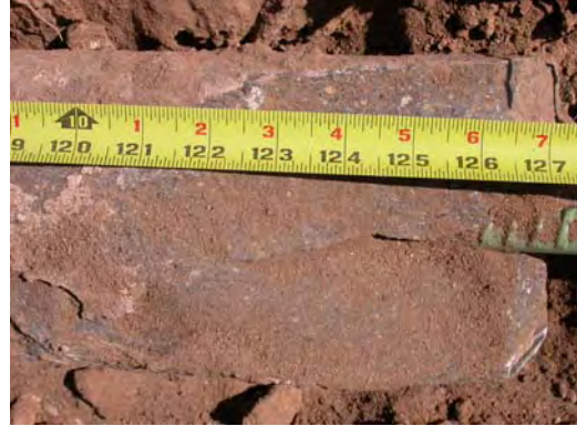
Grout ends at 10'7"
