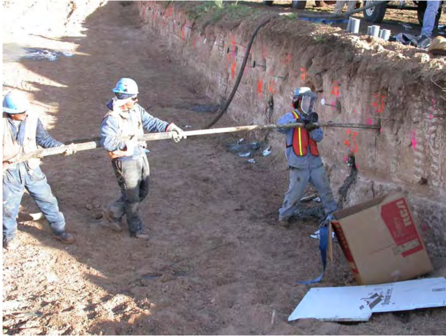
Figure 4.22 Soil Nail Grouting Using Tremie Pipe
