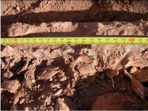
Partially grouted nail
