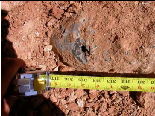
Grout goes through foam and ends at 26'5"
