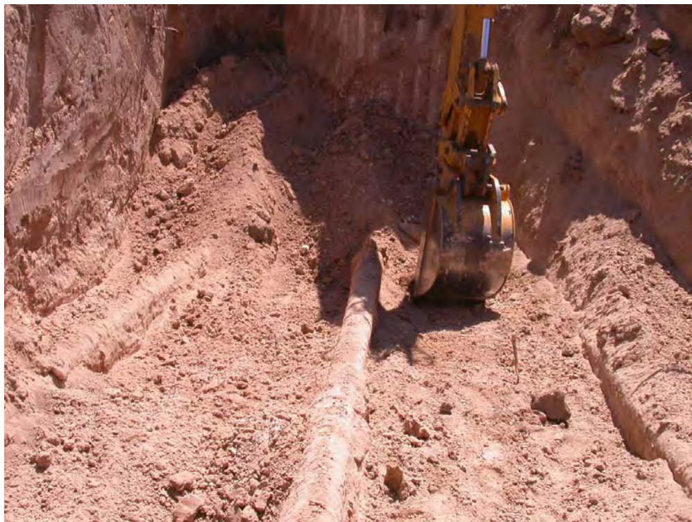
Figure 5.26 Backhoe Excavation Closer to the Nails
