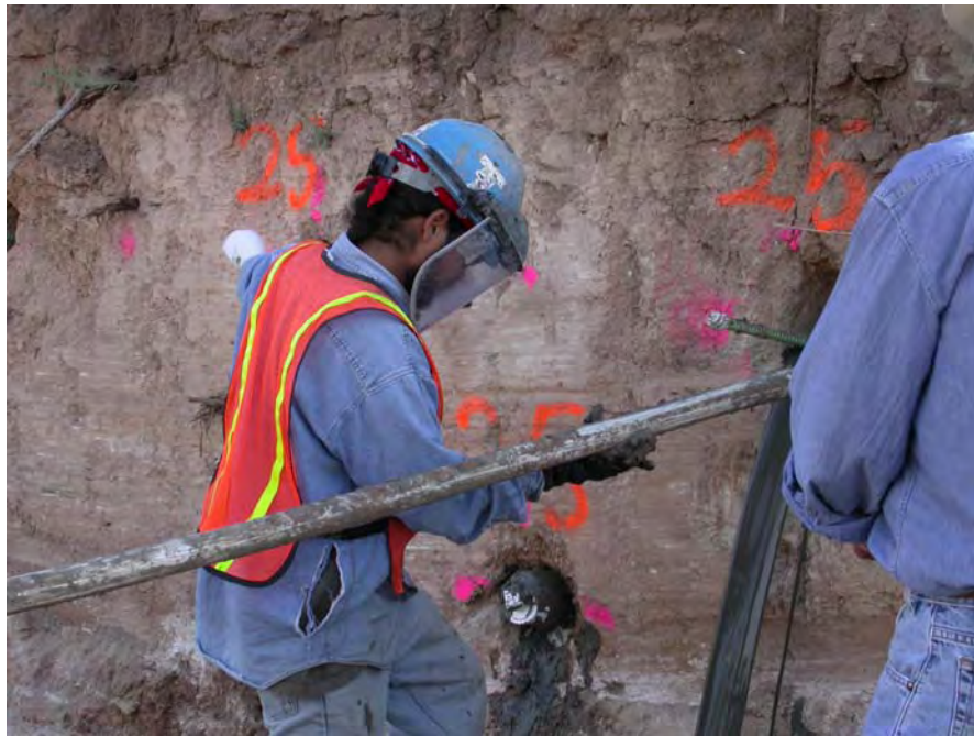
Figure 4.23 Grout Overflow at the Completion of Grouting
