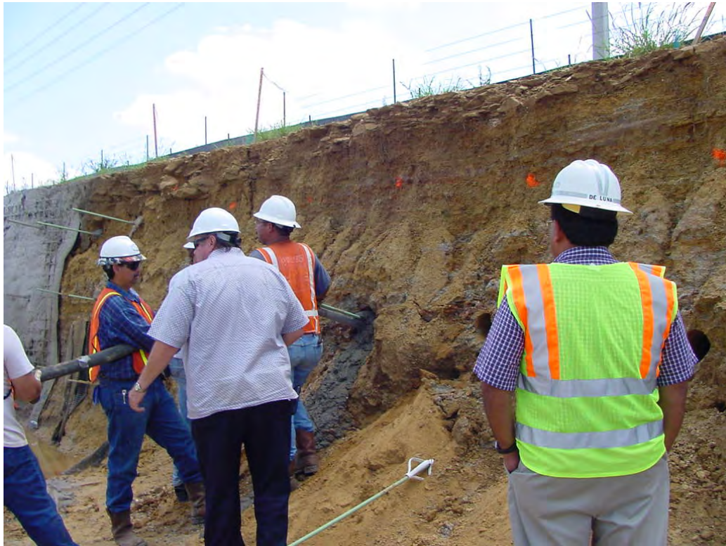
Figure 2.23 Inspection of Soil Nail Installation
