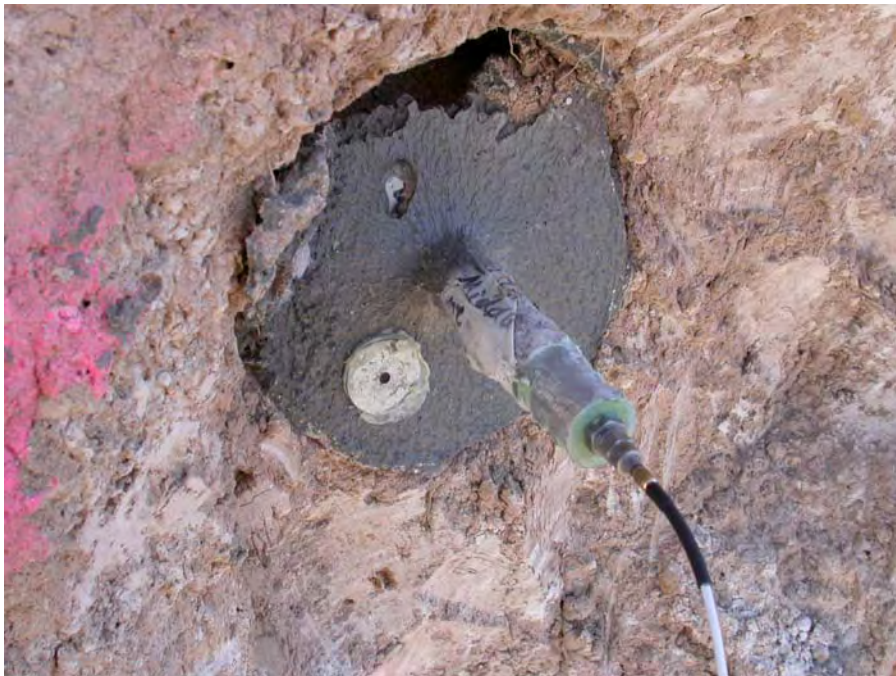
Figure 5.11 Grease was Used to Glue the Washer with the Grout
