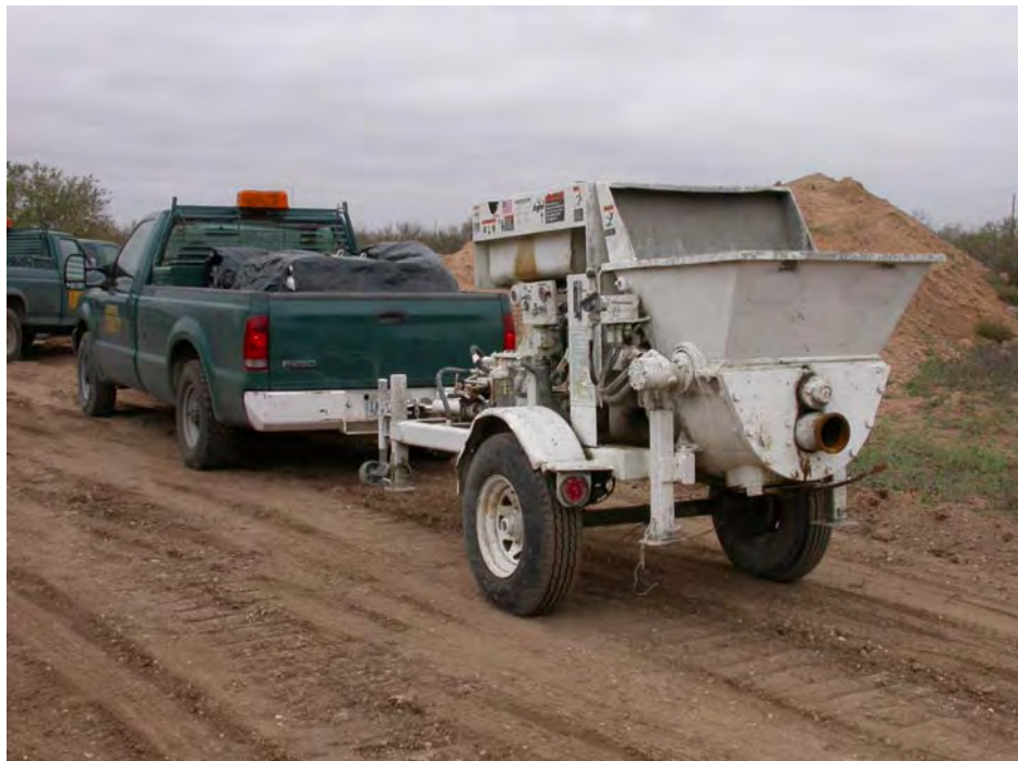
Figure 4.19 Grout Pump Used in Test Wall Construction
