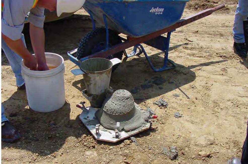
Figure 2.18 Stiff Grout Causes Incomplete Grouting Problem
