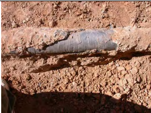
Grout goes through foam
