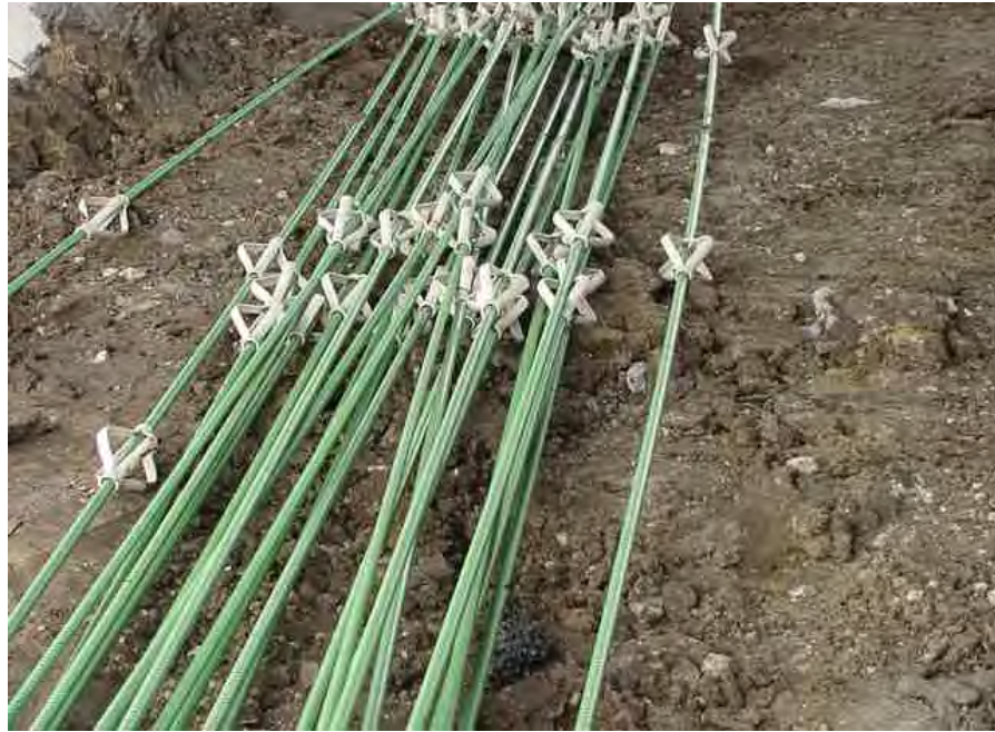
Figure 2.3 Epoxy-Coated Steel Tendons Used in TxDOT Installations
