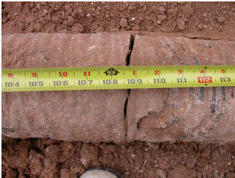
Figure 5.50 A Crack on Nail No. 5 at 9ft
