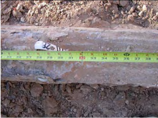
Partially grouted nail
