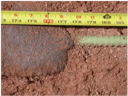
Grout ends at 14'9"
