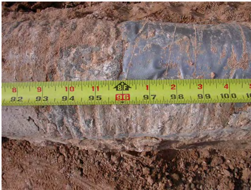
Figure 5.44 Nail No.16 Grout Meets the Foam at 8 feet and Passes Underneath
