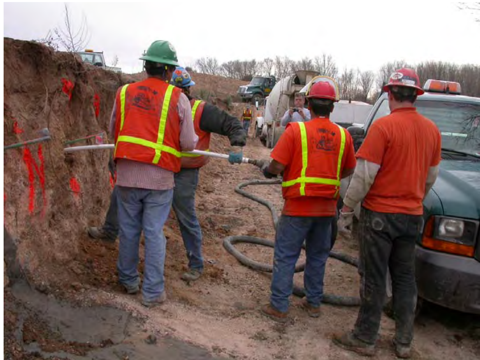
Figure 4.37 Grouting Nail No. 29 with the 20 feet Long Tremie Pipe
