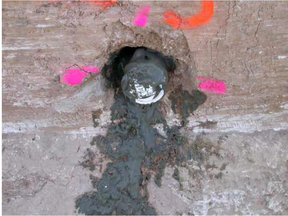
Figure 4.26 PVC Access Tubes after Annulus had been Grouted with Bentonite
