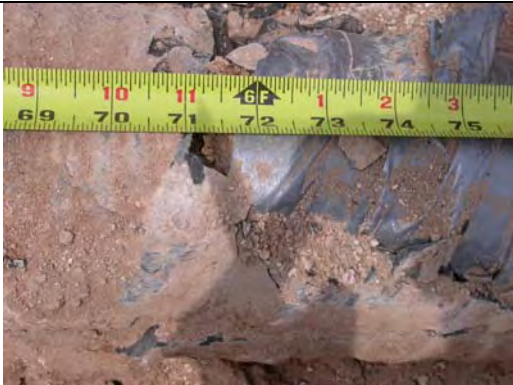
Grout passes through foam
