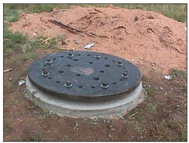
Figure 3.5 Foundation with Steel Plate
