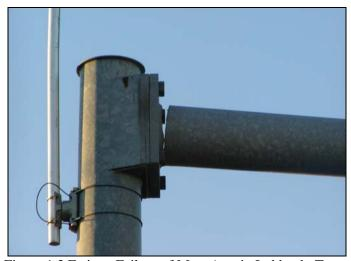
Figure 1.3 Fatigue Failure of Mast Arm in Lubbock, Texas
