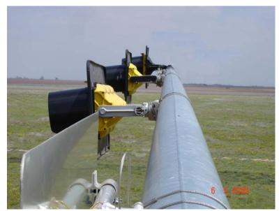
Figure 7.1. Traffic Signal Configuration Susceptible to Vortex Shedding
