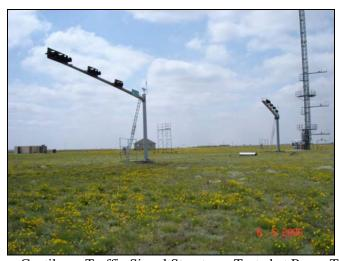
Figure 3.1 The Two Cantilever Traffic Signal Structures Tested at Reese Technology Center
