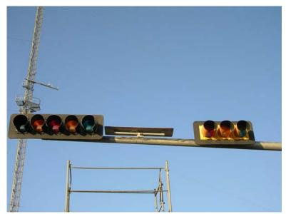
Figure E. 23 Mast arm with damping plate
