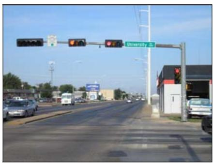
Figure 1.1 Cantilever Traffic Signal Structure with Straight Mast Arm
