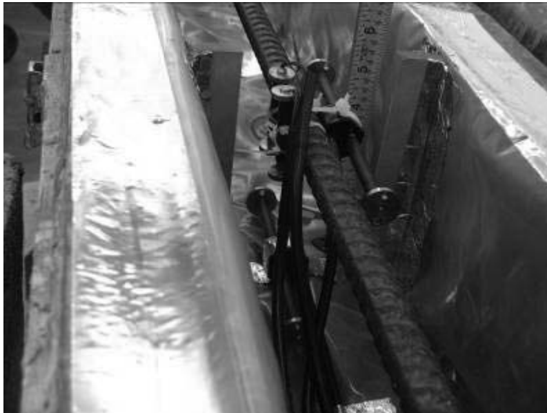
(b) Installed VWSGs
