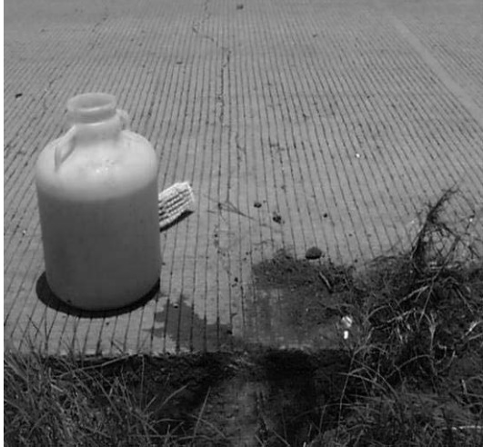
Figure 2.5: Horizontal cracks observed on the side of the slab
