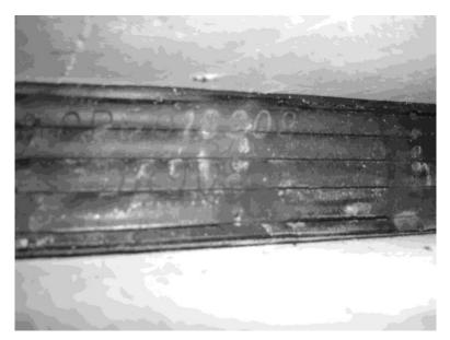
Figure 5.74 – Heavy Surface Cracking on an Elastomeric Bearing
