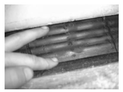
Figure 5.75 – Tension Debonding at Shims
