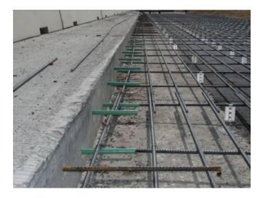
Figure 2.2: Tied and doweled sections
