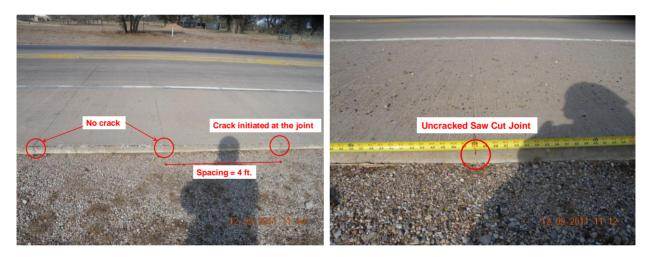
Figure 5.34 Cracked and Uncracked Saw Cut Joints in Abilene Whitetopping Section (SH 226 at SH 279)
