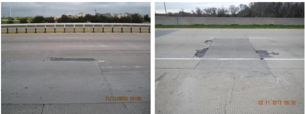
a. PCH-RJ (IH 30, Dallas District) b. PCH-RJ (IH 30, Paris District) Figure 2.23 Punchout at Repair Joint (PCH-RJ)
