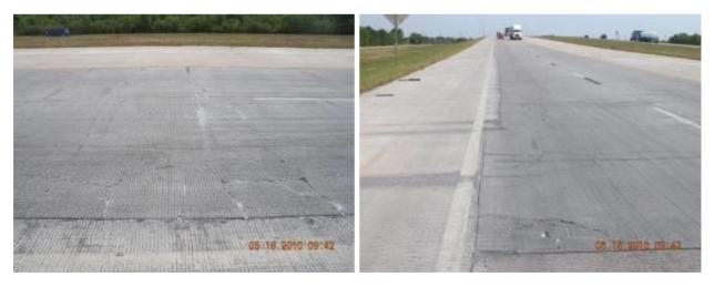
**Figure 5.25 Delaminations in BCO**
