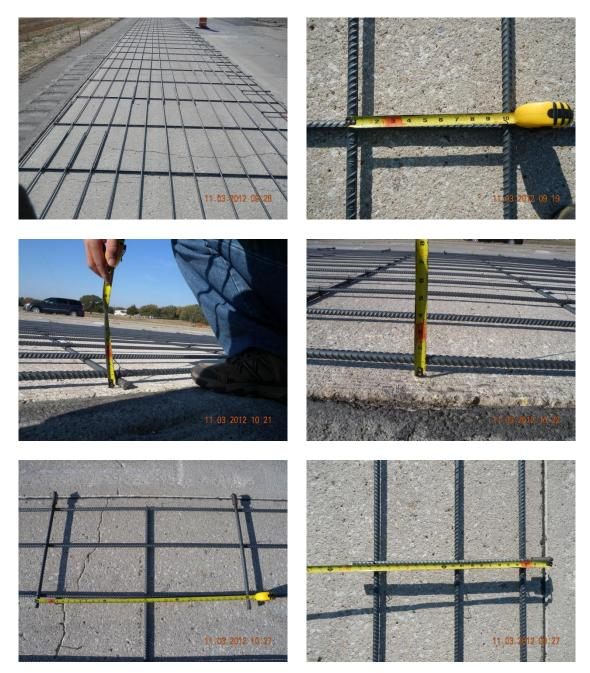
Figure D.3 US 287 Pavement Evaluation in the Wichita Falls District – Steel Placement (11/03/2012)
