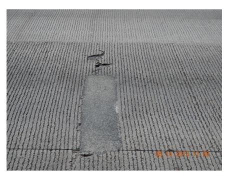
Figure 4.8 Close-Up View of Spall Repairs
