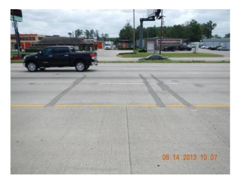
Figure 4.14 Spalling Repairs in SRG Section
