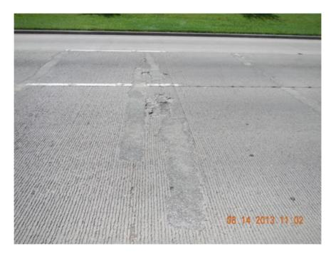
Figure 4.7 Deep Spalling in SRG Section
