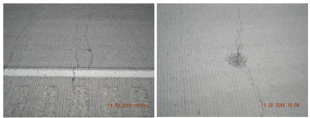
Figure 4.33 Transverse Cracks in Van Horn Figure 4.34 Spalling Distress in Van Horn IH IH 10 10
