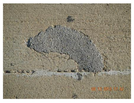
Figure 5.14 Asphalt Concrete Patch at Joint (North)
