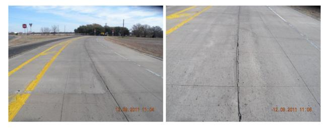
Figure 5.32 Whitetopping in Abilene (SH 226 at SH 279)
