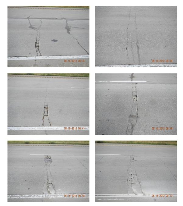
Figure D.6 IH 35 Pavement Evaluation in the Laredo District – Pavement Condition (05/15/2012)
