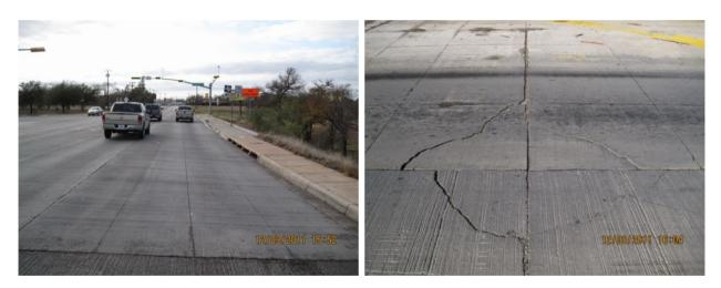
Figure 5.30 Whitetopping in Abilene (SH 36 at FM 1750)
