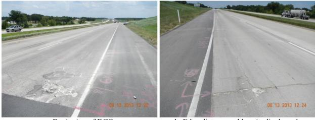
a. Beginning of BCO b. Edge distress and longitudinal crack Figure 5.20 Distresses in BCO
