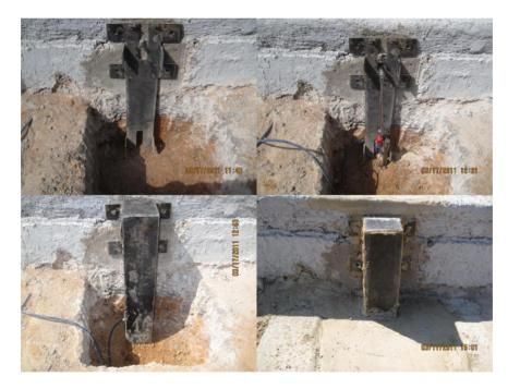
**Figure 3.1 Crackmeter Installation**
