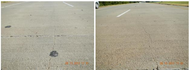
a. Longitudinal crack (outside lane) b. Longitudinal crack (inside lane) Figure 5.13 PCP in Georgetown (North)
