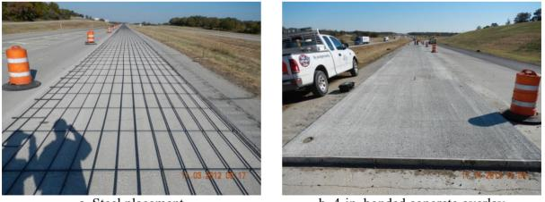
a. Steel placement b. 4-in. bonded concrete overlay Figure 5.18 4-in BCO construction
