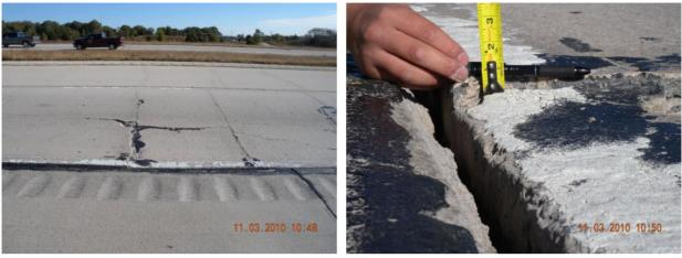
a. Typical edge punchout b. Joint separation and slab settlement Figure 2.20 E-PCH (US 287, Wichita Falls District)
