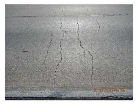
Figure 2.18 Y-Crack and Narrow Crack on US 81 in the Wichita Falls District
