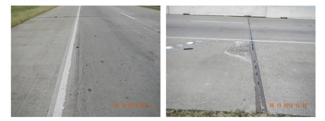
Figure 5.6 Longitudinal Cracks (built in 1985) Figure 5.7 Joint Failure in Shoulder (built in 1985)
