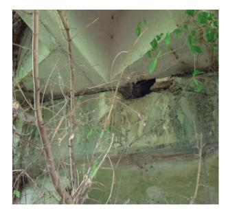
Figure 2.11 Damage in bent cap
