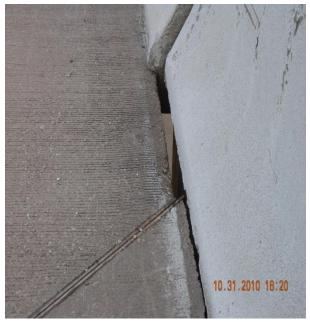
Figure 2.14 Misalignment of traffic rail (2)
