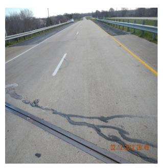
Figure 2.18 Transverse cracks near armor joint
