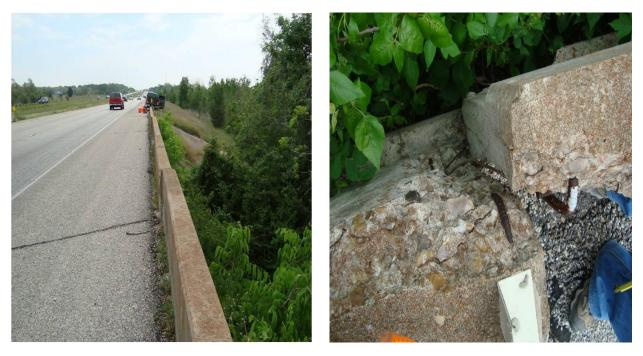
Figure 2.9 Misalignment of the traffic rails
