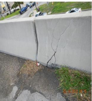
Figure 2.8 Damage in traffic rail
