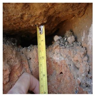
Figure 2.20 Void under bridge approach slab
