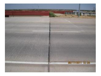
Figure 5.6 Expansion joint at the west end of the CRCP
