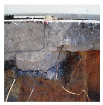
Figure 2.23 Expansion joint with support slab
