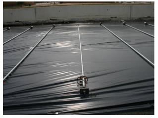
Figure 4.56 Polyethylene sheet placed between subbase and CRCP
