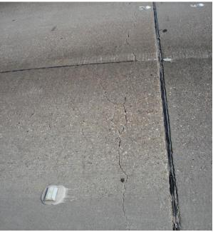
Figure 2.22 Transverse cracks due to voids
