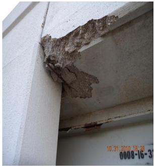
Figure 2.16 Damage in the bridge superstructure
