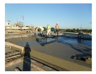
Figure 4.53 Concrete placement on the AL
