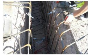
Figure 4.49 Installation of VWSGs in AL1
