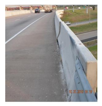
Figure 2.13 Misalignment of traffic rail (1)
