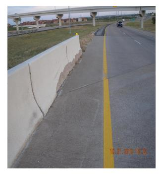
Figure 2.15 Damage in traffic rail
