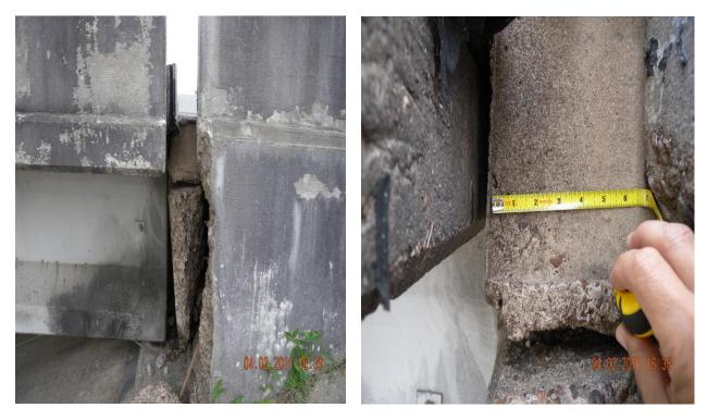
Figure 2.1 Damage in the abutment
