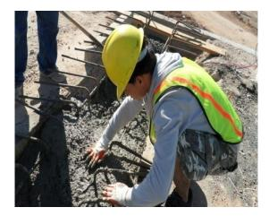
Figure 4.52 Covering the gages with concrete
