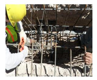
Figure 4.50 Installation of jackout pressure cells
