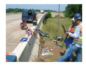
Figure 4.31 Location of crackmeter installation
