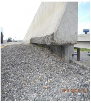
Figure 2.6 Subsidence of embankment material (1)
