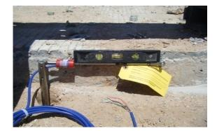
Figure 4.14 Installation of the crackmeter
