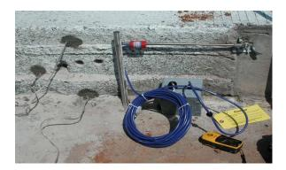
Figure 4.18 Installation of the crackmeter
