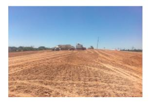
Figure 4.41 Subbase type 6 inches CSB
