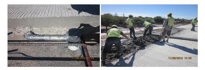
Figure 4.54 Crackmeter installation with protection
