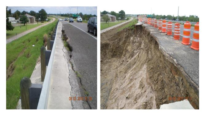
Figure 2.3 Slope failure in the embankment area
