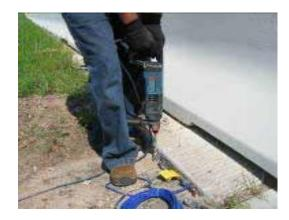
Figure 4.2 Drilling of a vertical hole to install invar
