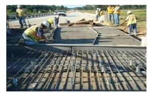
Figure 4.23 Finishing of the concrete
