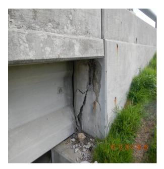
Figure 2.17 Damages in abutment
