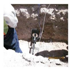
Figure 4.10 Installation of pressure cell in the AL
