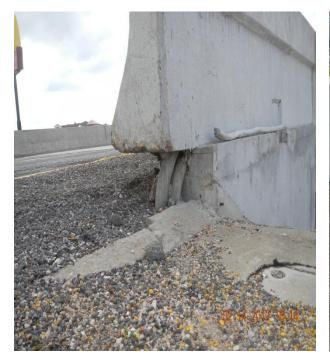
Figure 2.7 Subsidence of embankment material (2)
